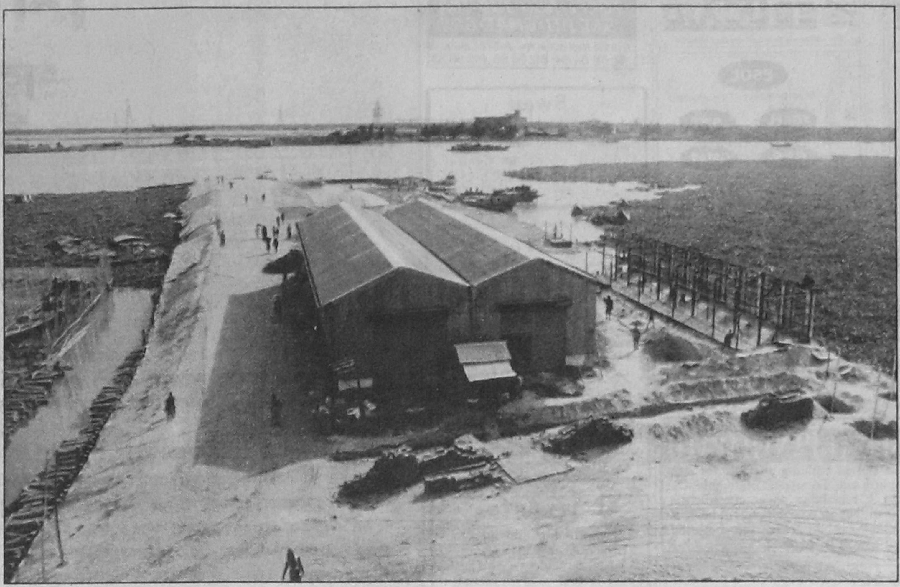
The Sena Kalyan Sangstha (SKS) establishment on the river Buriganga. This is the photograph of the Sangstha's storage facilities, taken on Wednesday showing encroachment of the river. We inadvertently published the photograph of another illegal structure describing it as a SKS establishment. We regret the mistake but will publish the story of that illegal construction very soon.
