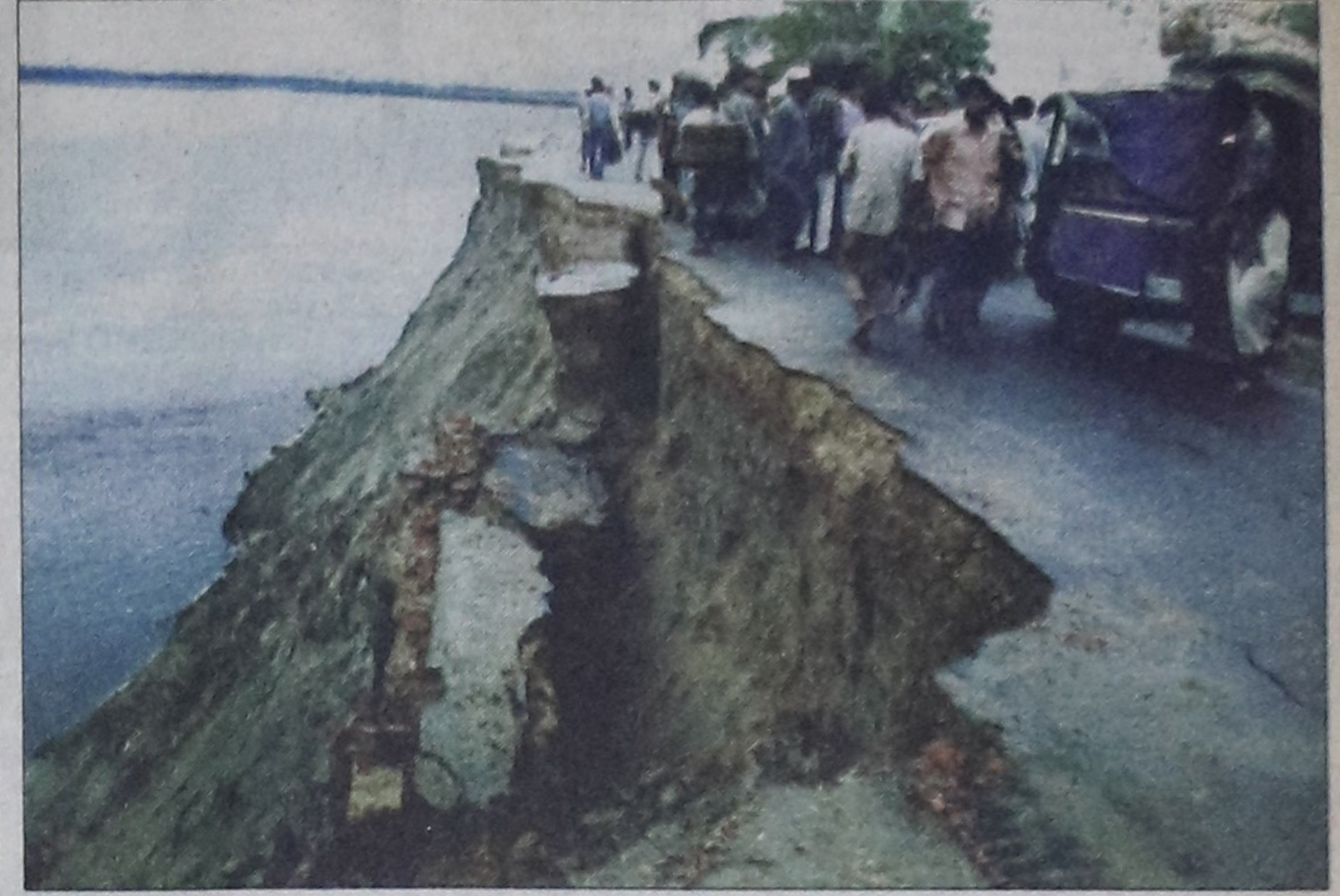
A river retaliates: Direct road link between Jamalpur and Sherpur has been suspended since June 2 thanks to unabated erosion by the old Brahmaputra. The reason has been put down to change of course of the river caused by closure of one of its channels last year, leaving the ferry ghat most vulnerable.
