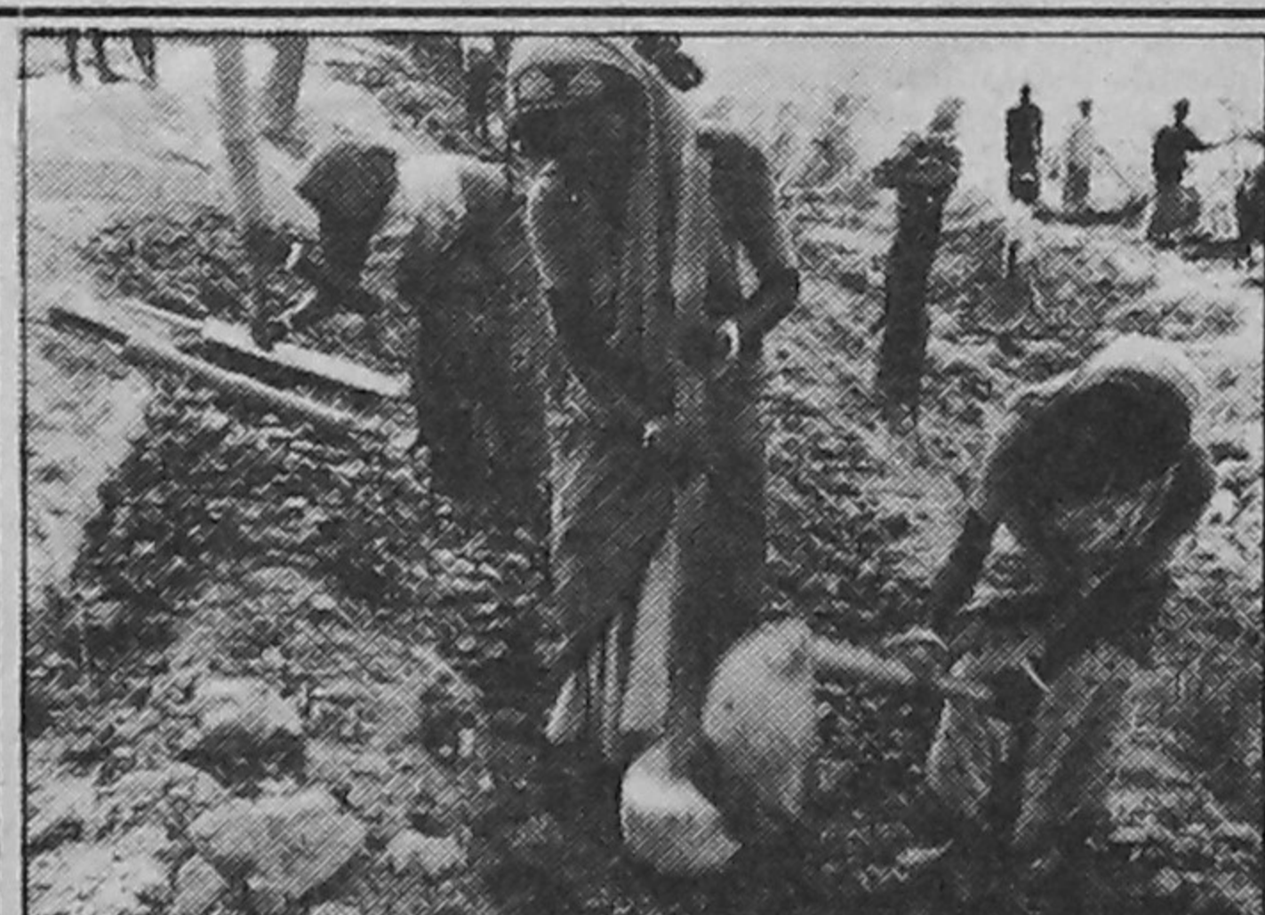
Labour Contracting Society (LCS) members engaged in embankment compaction
