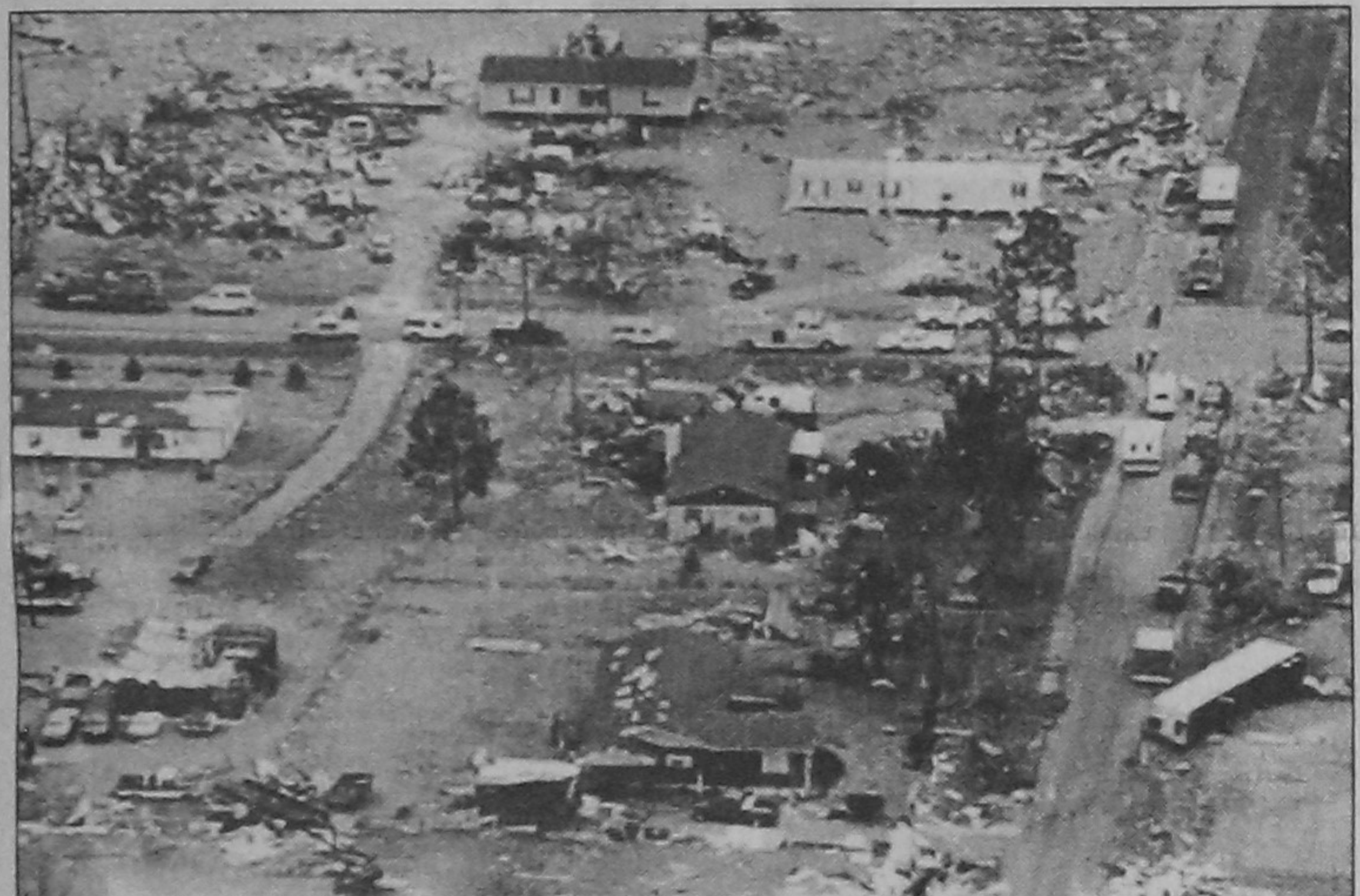
A housing development lies in ruins following a tornado in Camilla, Georgia. Tornadoes slashed through southwest Georgia early Monday, killing at least 22 people and injuring more than 100. — AFP photo
