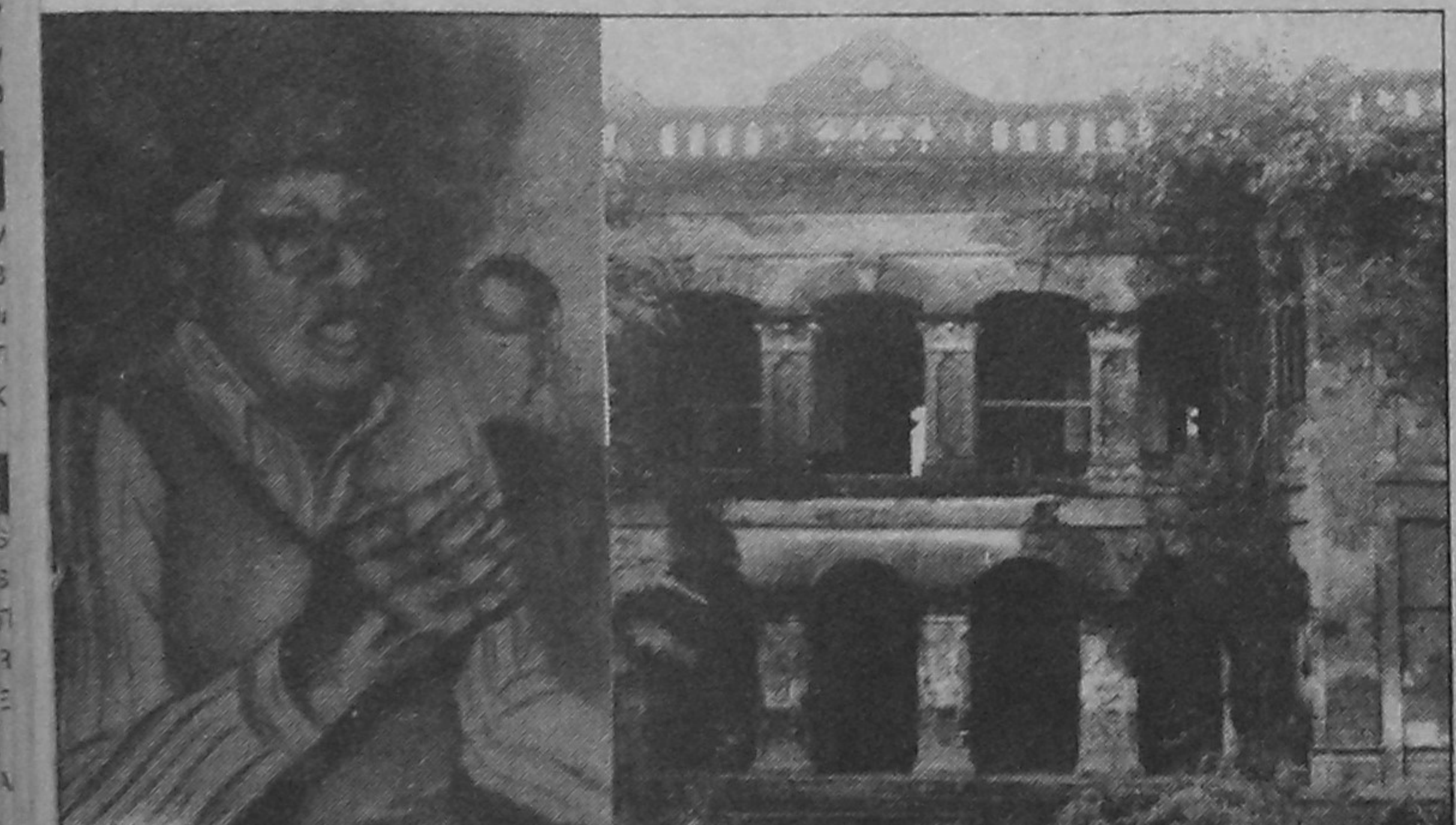
(L-R): Kazi Kader Nawaz and his residence which is now in dilapidated condition at village Muzdia in Sreepur thana of Magura district. — Star photo
