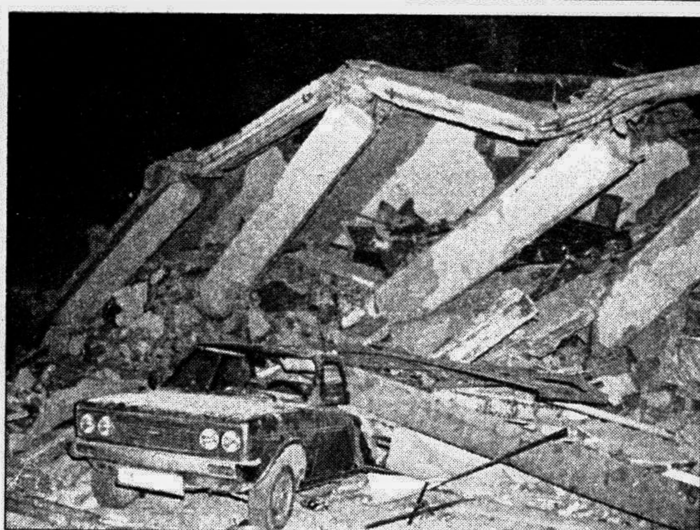
A vehicle was crushed under the weight of a collapsed building in Bolu, north-western Turkey in the early hours of Friday during a strong earthquake that was felt across the country. The epicentre of the 7.2 quake was near Duzce where the death toll already crossed 300 yesterday. — AFP photo
