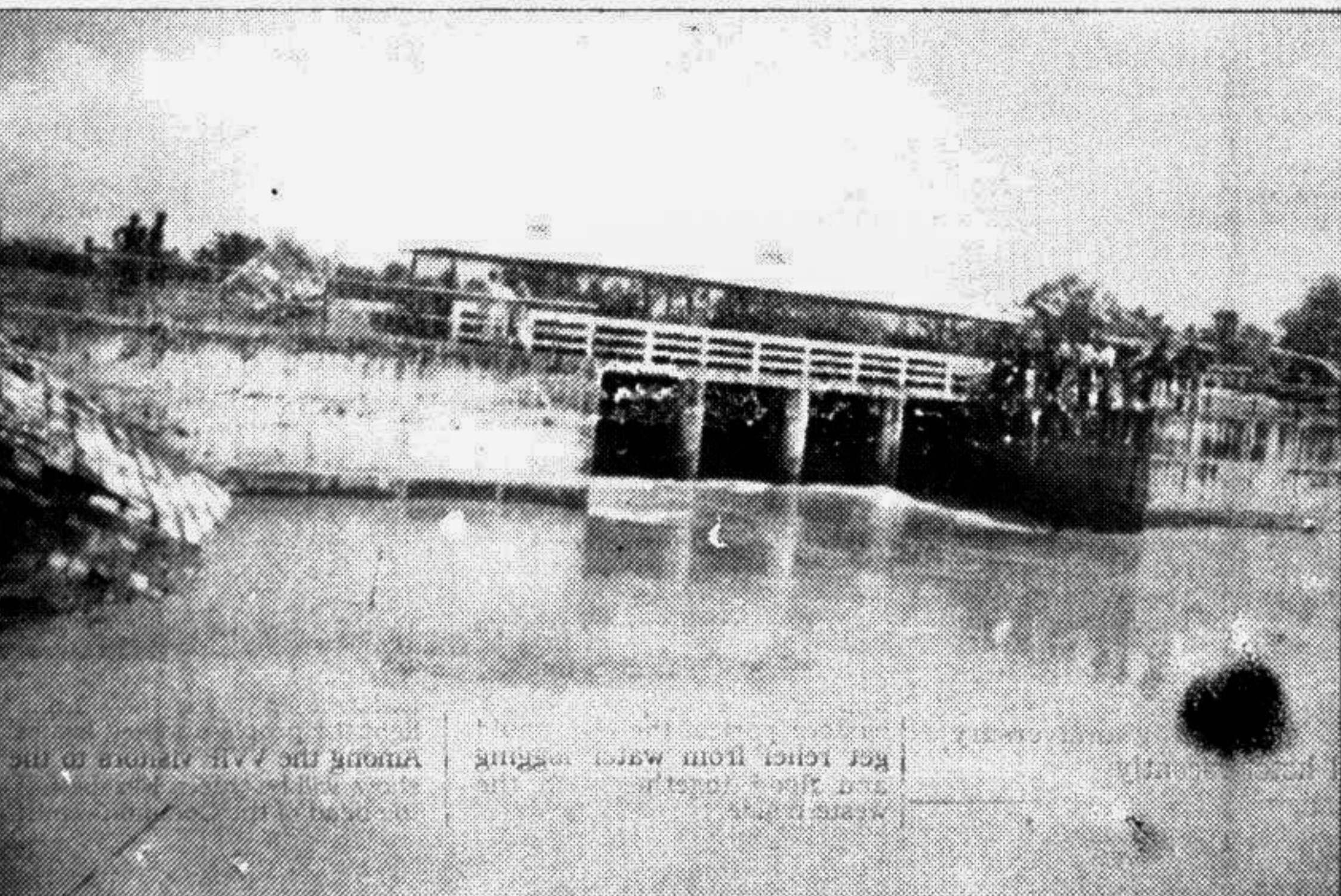
Natore district office of Bangladesh Water Development Board (WDB) has launched a massive riverine structural development scheme named Baral Dam Development Project involving Taka 17,57,40,000. The scheme has been aimed at protecting 1.10 lakh hectares of crop lands from the fury of flood and bringing drought prone crop lands under the irrigation network. WDB has constructed two power dam regulators with a capacity of 5,000 cusec each at Charghat and Atghoria, 16 km away, cum flashing sluice gates during the period of 1994-98. Photo shows the Atghoria regulator at the connecting point of the Baral and Nandabuzha. —Star photo
