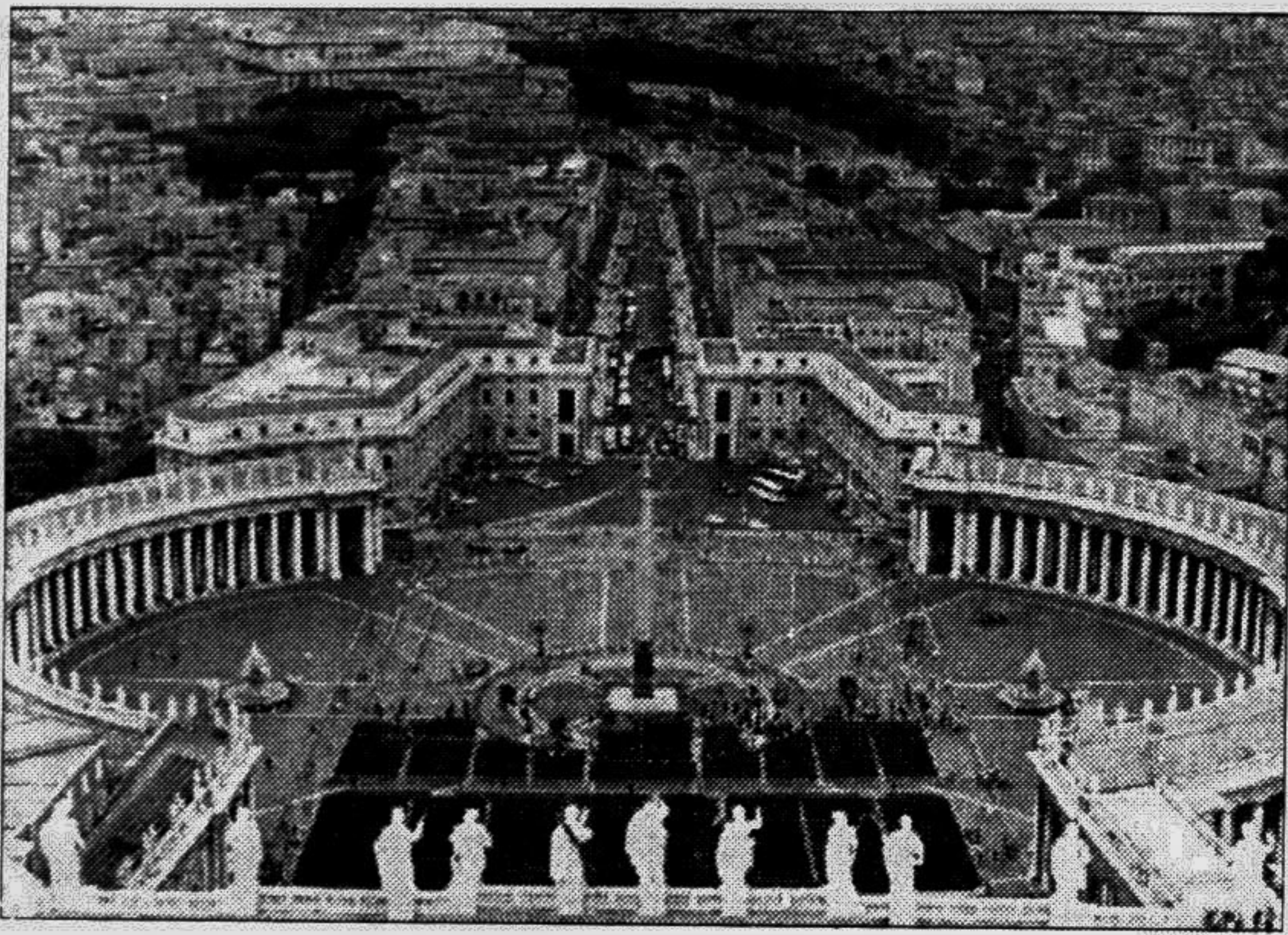
This photo, taken from the dome of Saint Peter's, shows the size and shape of Saint Peter's square. Built in 1667 and designed by Bernini, the square is enclosed by a grand colonnade that consists of three aisles between four rows of columns. By a trick of visual perspective, a tourist standing on a stone marker near the Egyptian obelisk sees only one row of columns — the other three rows line up perfectly behind the front column. The square can easily hold over 400,000 people. The broad street leading from the square, the Via della Conciliazione, was built by Mussolini in the 1930's and leads to a bridge across the Tiber River.
