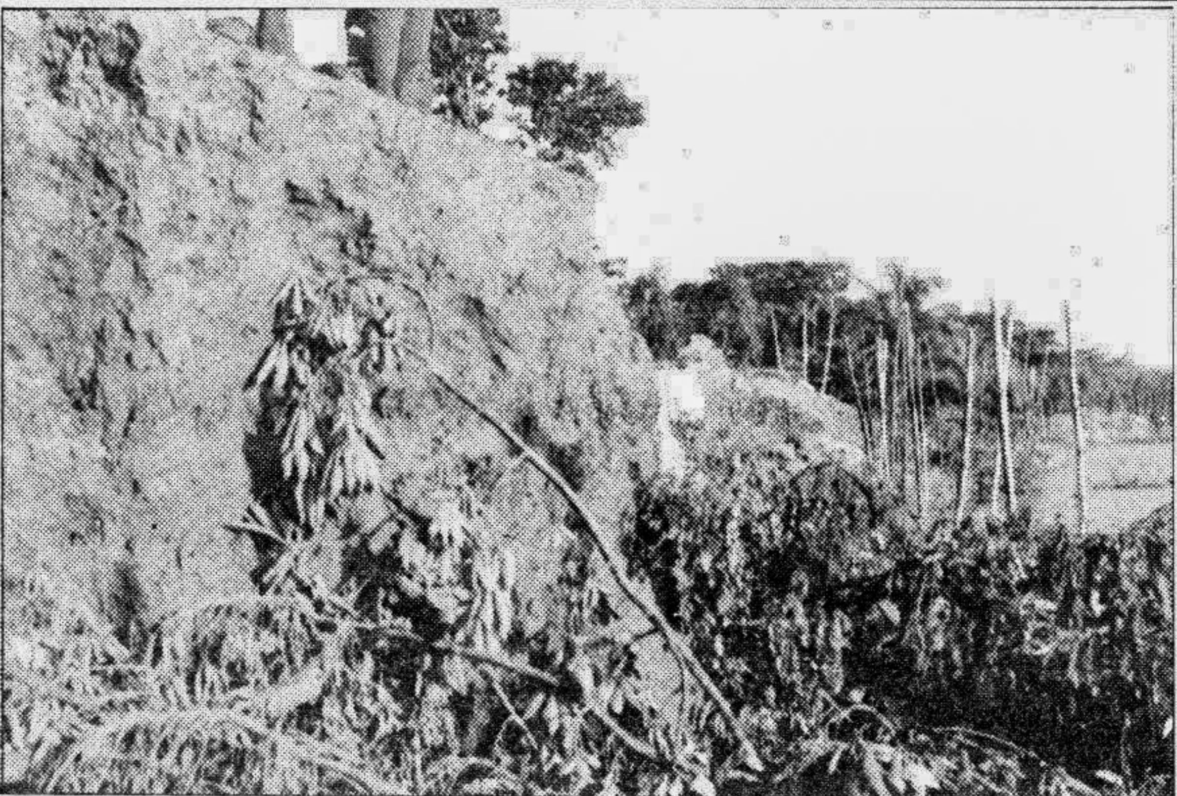
Checking erosion: Erosion by the Meghna in Chandrapur town is being checked by placing bamboos, trees, bricks and sand bags. — Star photo
