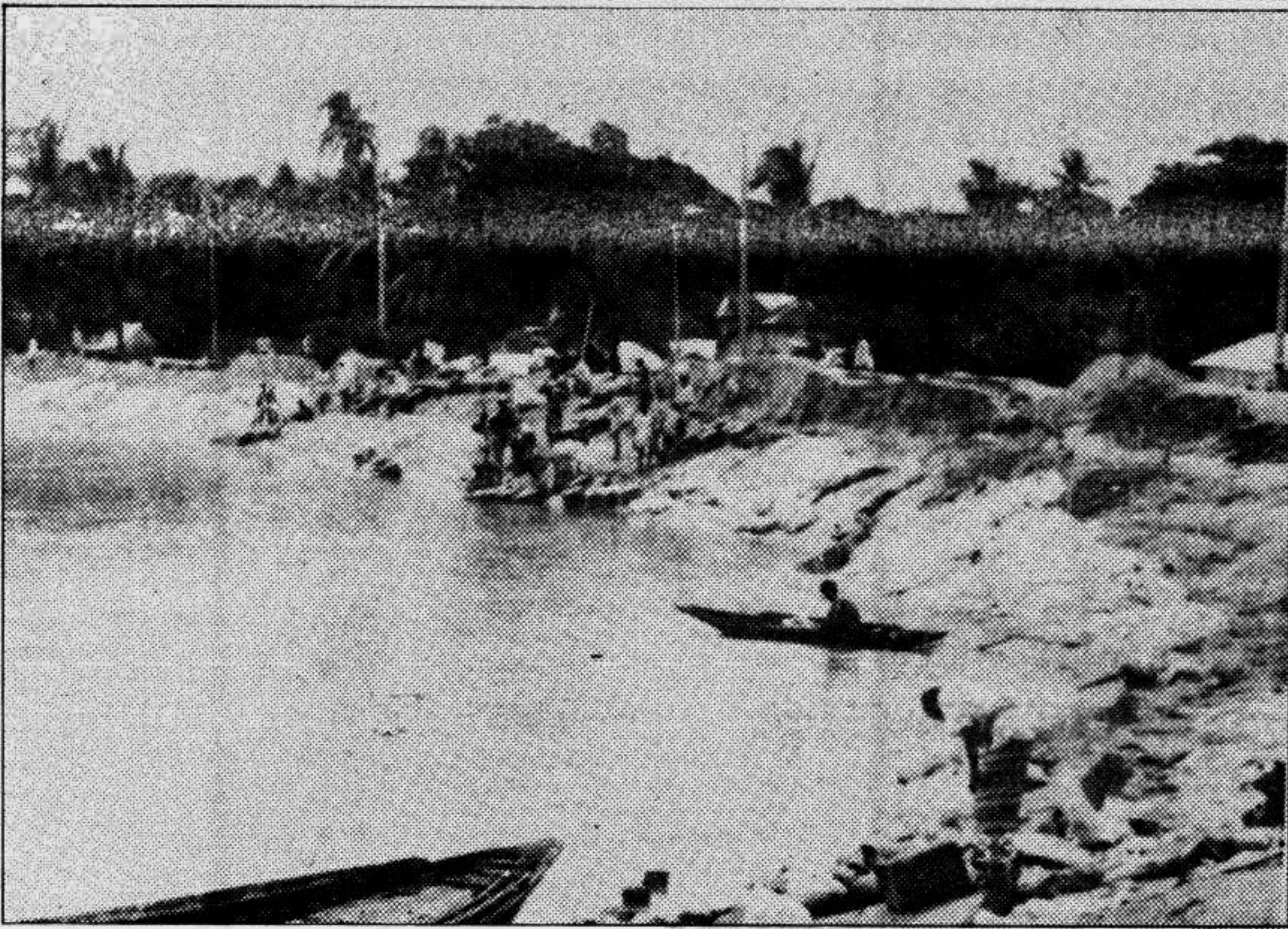
Haridashpur village has been partially damaged recently by the Modhumati erosion in Gopalganj. — Star photo
