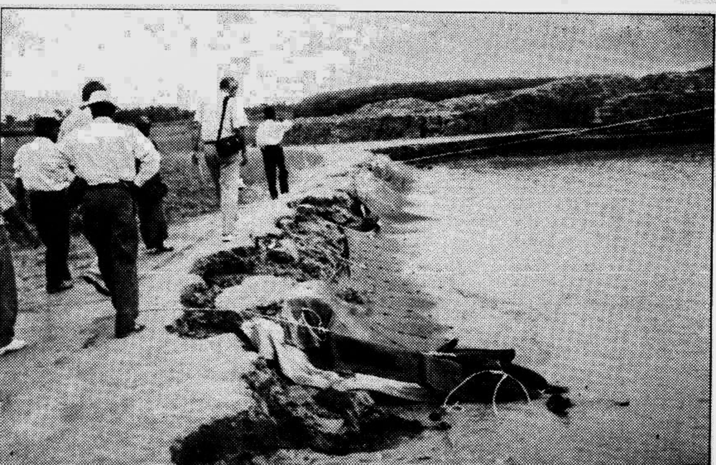
The Netherlands government has undertaken a scheme on experimental basis to check the erosion at Haimchar by placing geo-textile clothes on the eroded area. —Star photo
