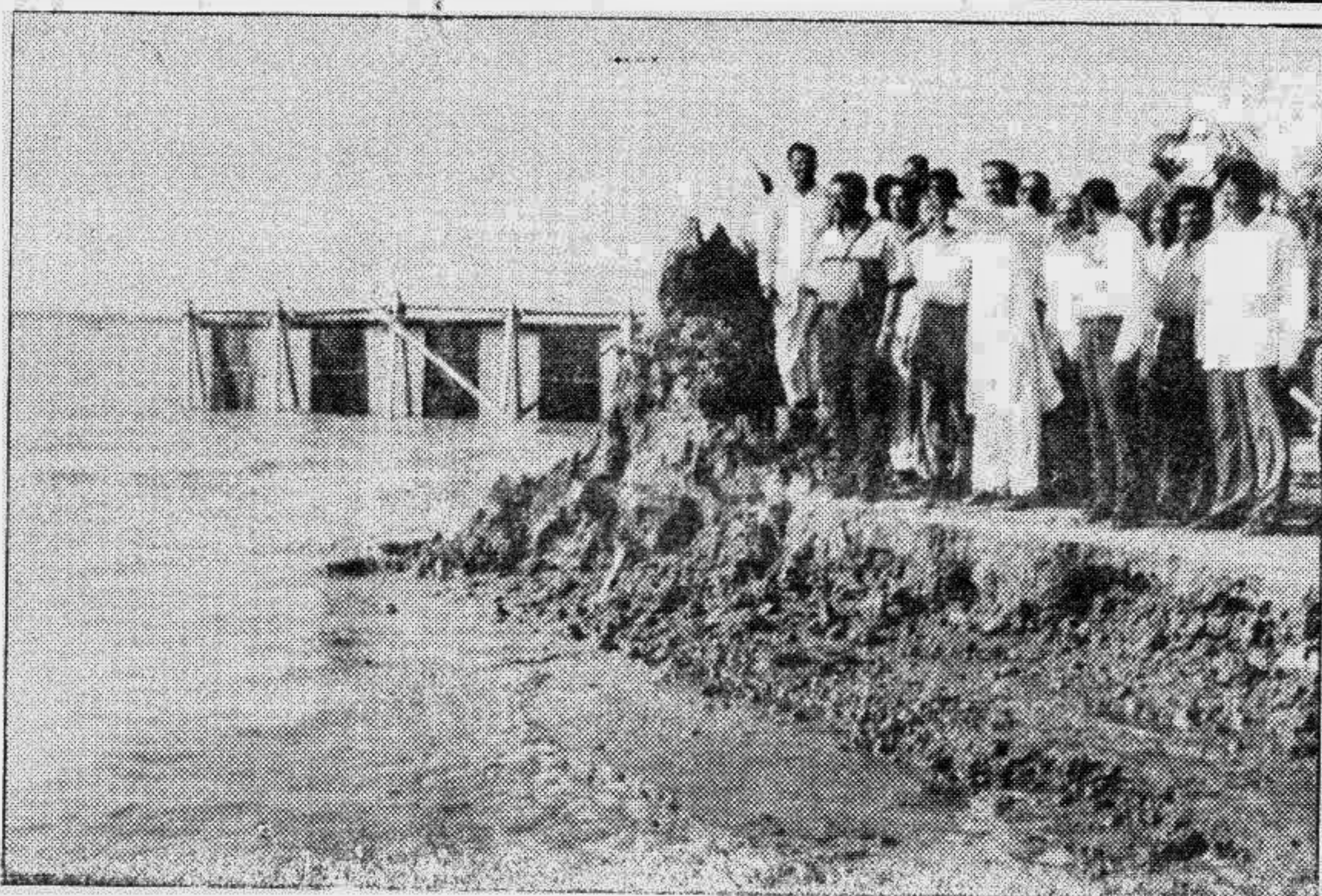
The endless onslaught: Md Rezaul Karim, deputy commissioner, Chandpur and Bangladesh Water Development Board officials visited the erosion affected areas of Haimchar thana. — Star photo
