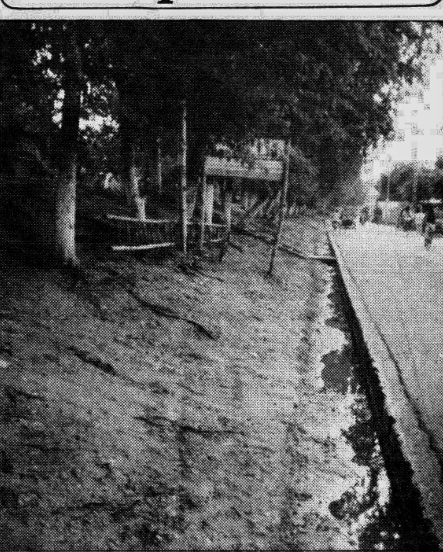
Trees are not always good: The RCC has planted hundreds of trees on the Rajshahi town protection embankment. Some experts feel that the trees are making the already vulnerable century old embankment weaker by spreading their roots in all directions.
