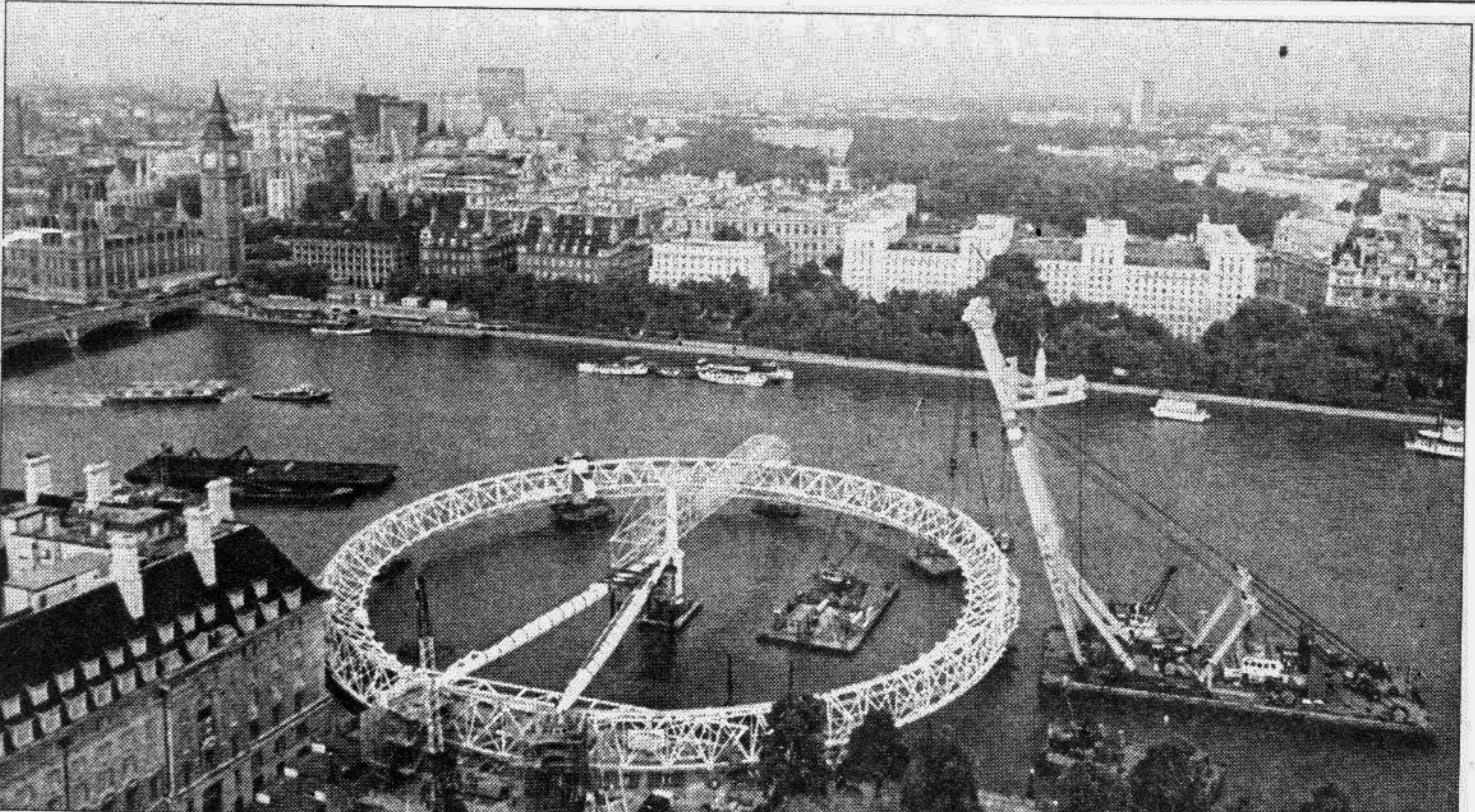
The final rim section of the British Airways London Eye big wheel is laid in place, encircling the newly installed hub and spindle and column, legs by London's County Hall, Tuesday. The British Airways London Eye will be open to the public in January 2000 offering 2.2m visitors a year unrivalled views of the city in a 30 minute trip. — AFP photo
