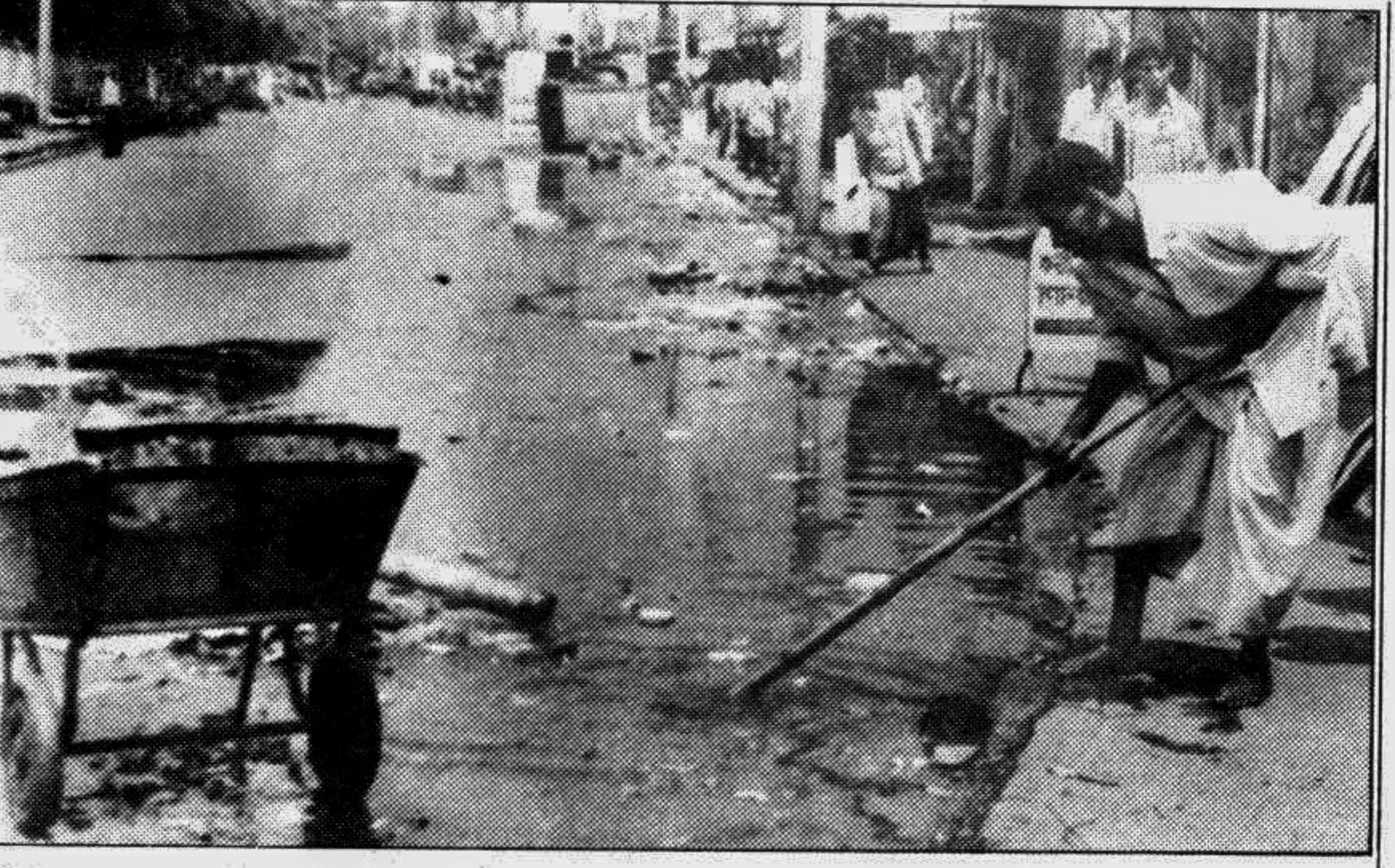
Filthy water submerges the roads due to faulty drainage system in the Ananda Bazar area in the city.
