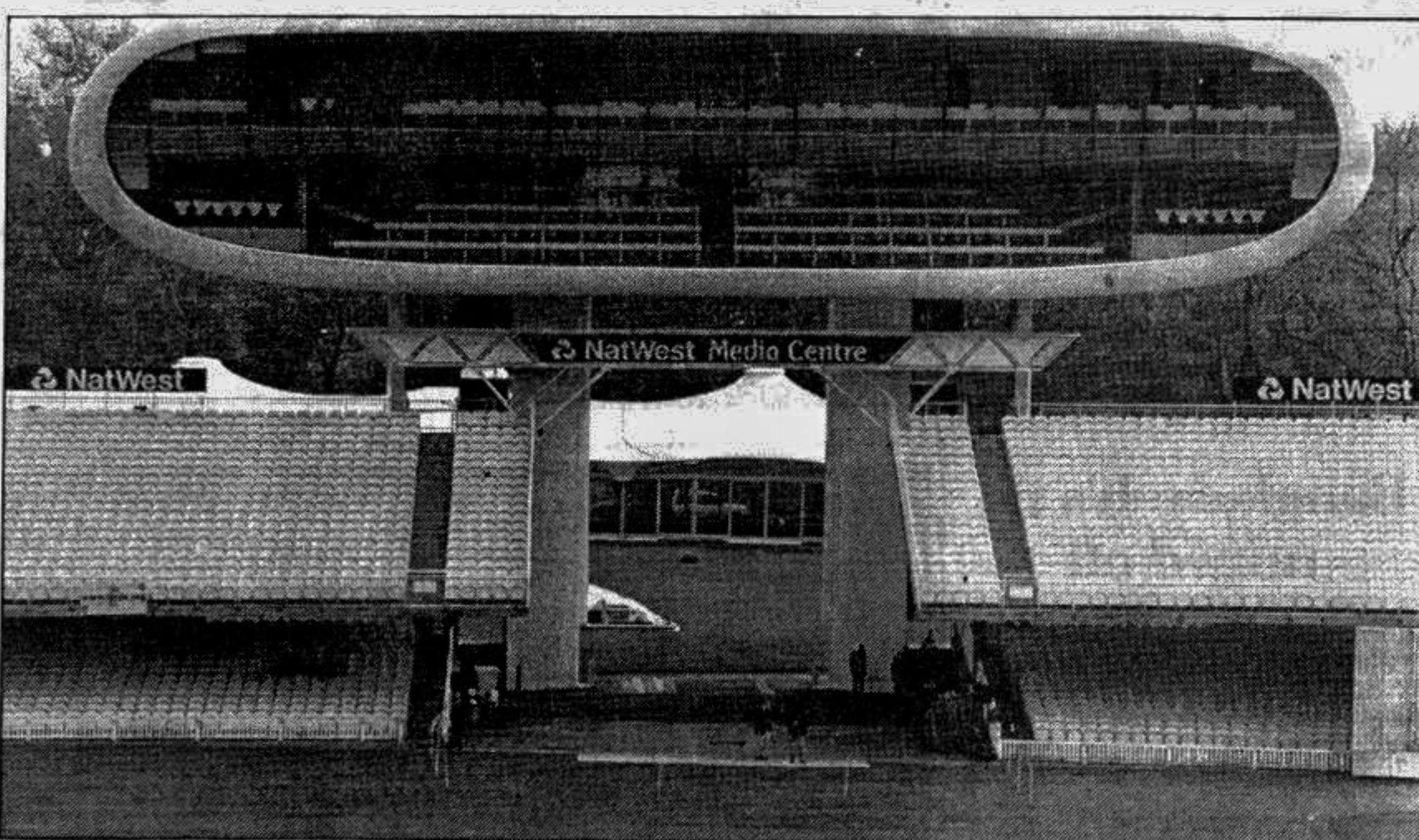
JUST LANDED! The new media centre at Lord's Cricket Ground in London, named 'Spaceship', was unveiled on April 27. The 5.8 million pounds structure will accommodate 250 pressmen.
