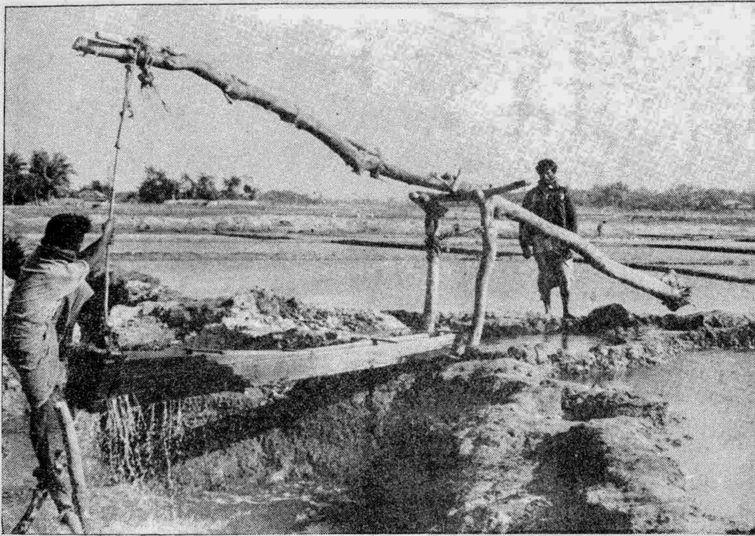
Channelling water from the sea to production area
