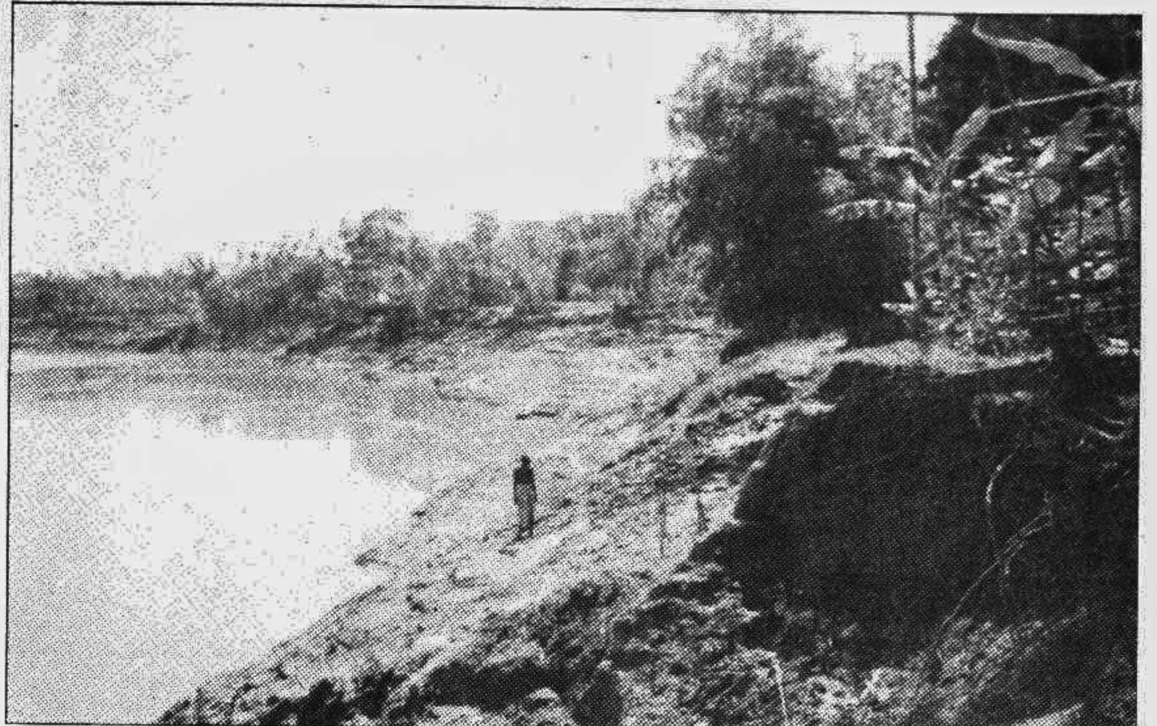
SYLHET: Erosion by the river Kushiara has taken a serious turn along several villages in Jakiganj thana. The erosion is reducing the country's territory for the last few years. Steps taken by the Water Development Board so far are not satisfactory. This photo was taken from village Gangajal. — Star photo by Iqbal Siddiquee
