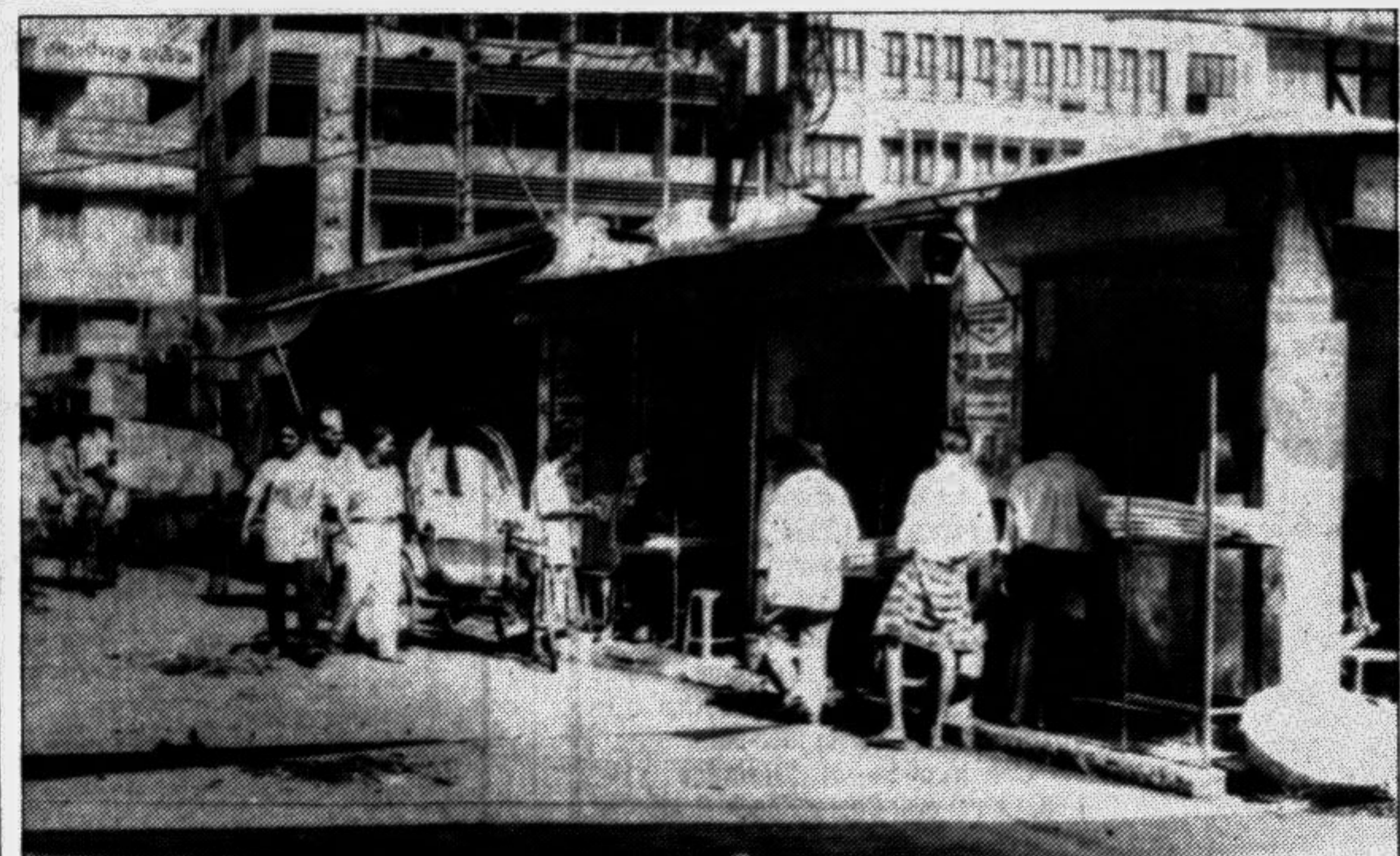
Shops have been set up illegally on public land and part of the road near Meillat office in the city's Fakirerpool area. Illegal structures are also being built on the land still vacant. — Star photo
