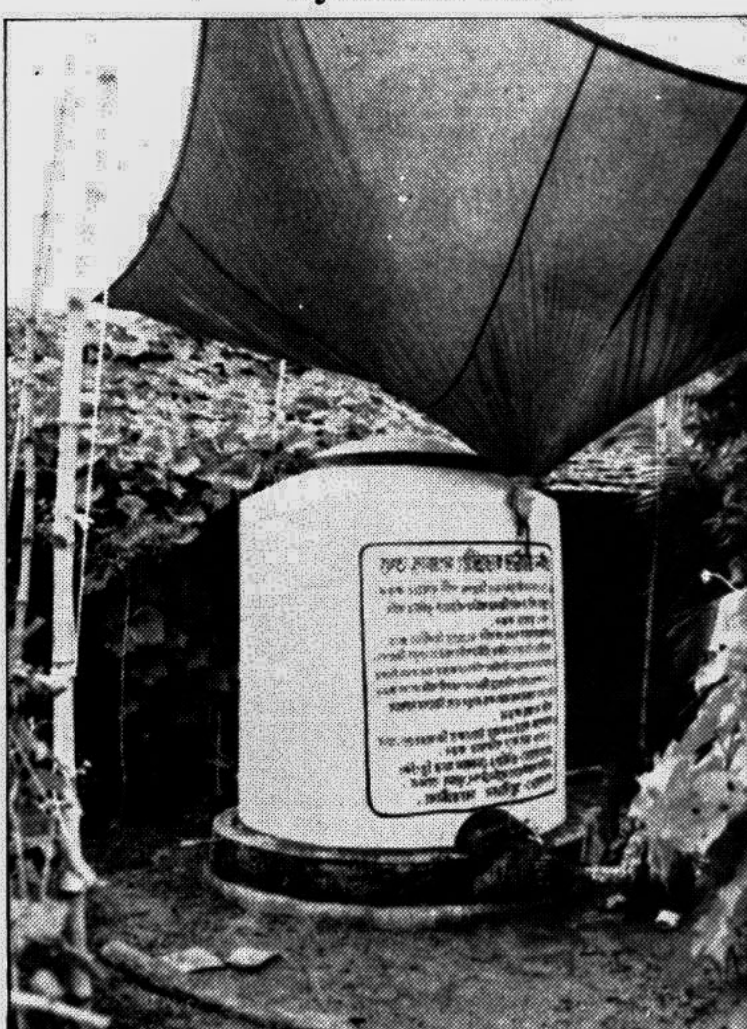
Azibur Rahman's Rain water Harvesting Plant
