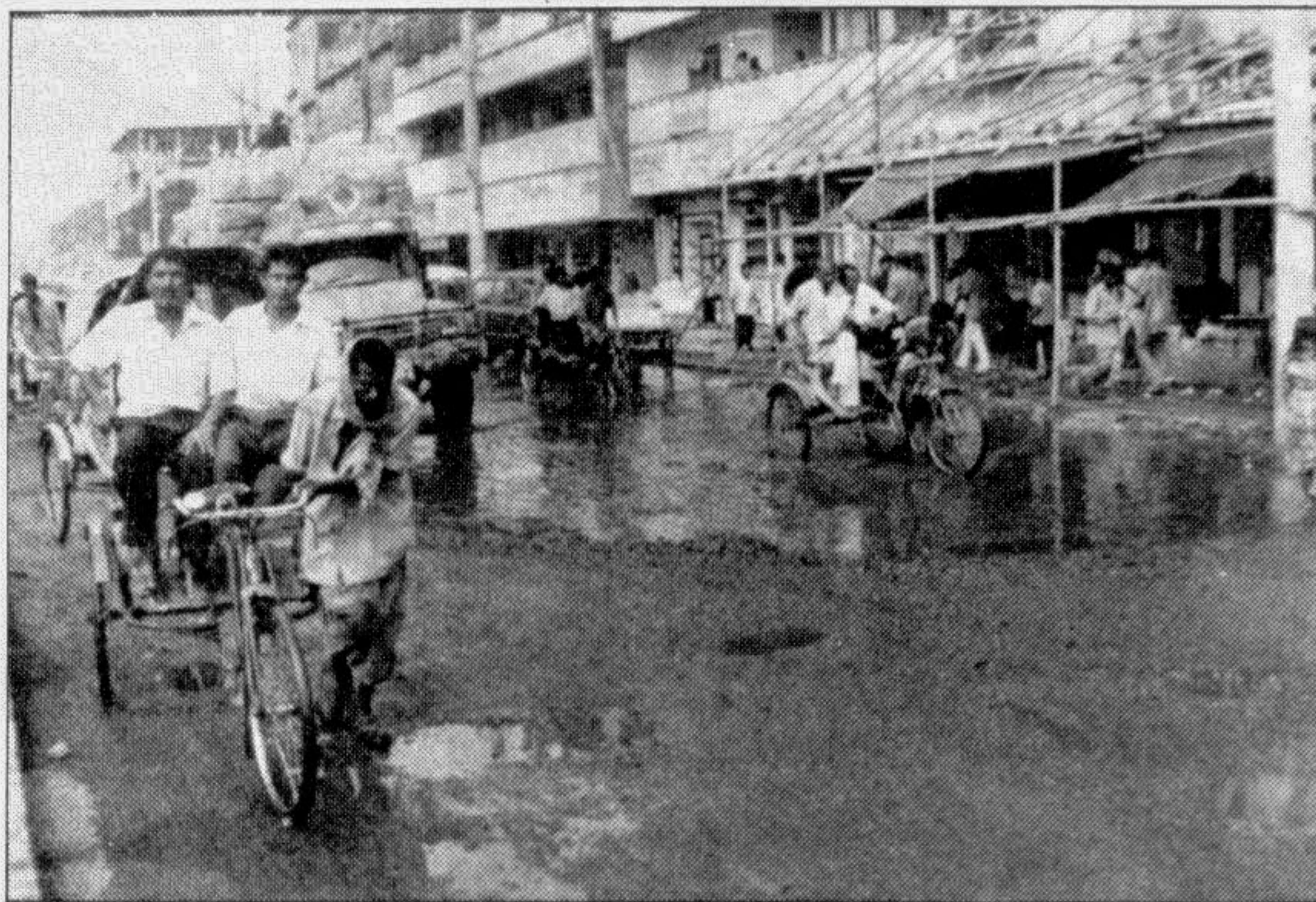
NARAYANGANJ: Floods have damaged the Chamber Road of the town causing immense sufferings to the town dwellers. Their woes multiply when rain water remains stagnant for days together in potholes of cracked roads. — Star photo by Ehsanul Haque
