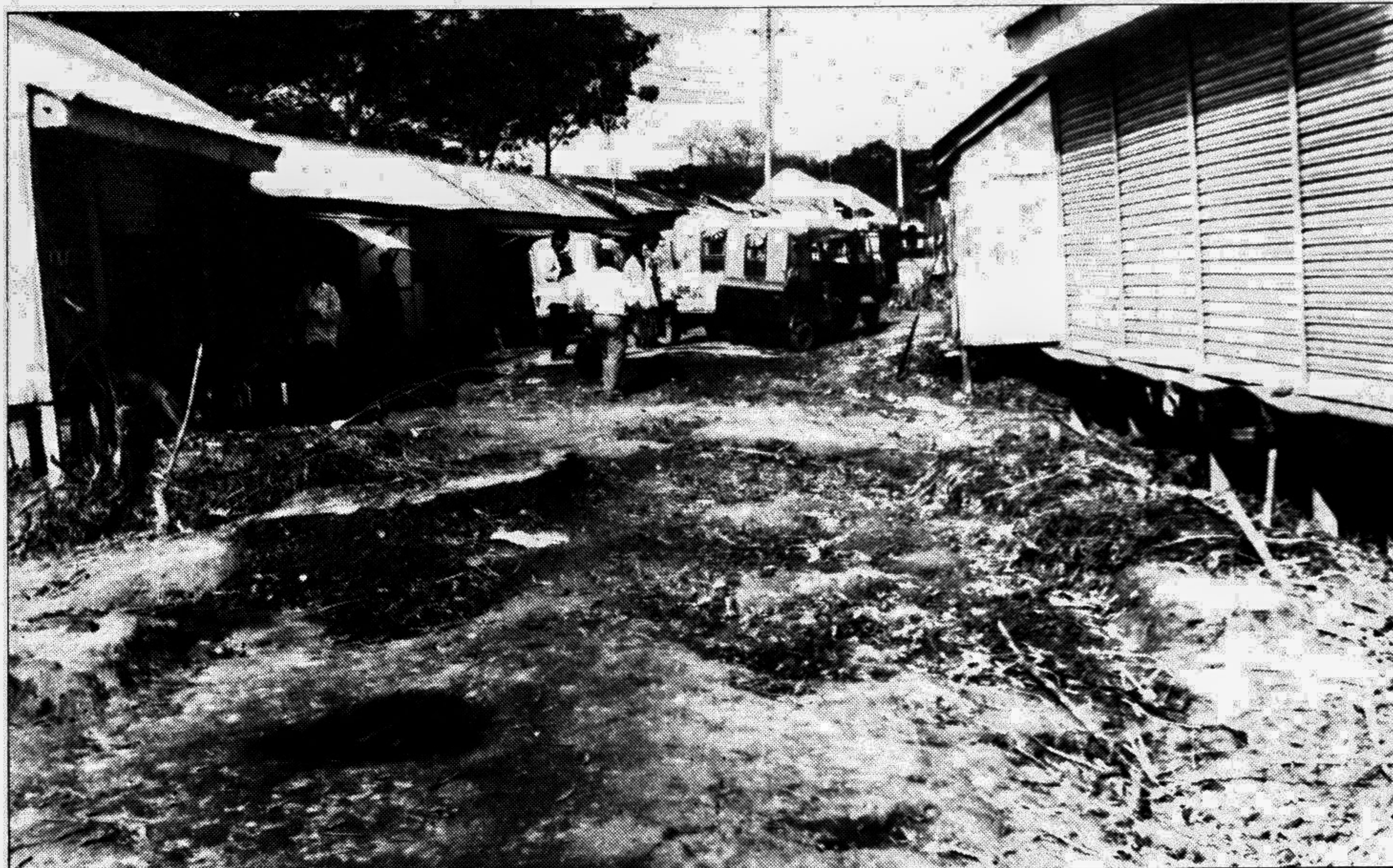
Chandar Bazar, Munshiganj; Flood water has receded taking with it the crust of the road away.
