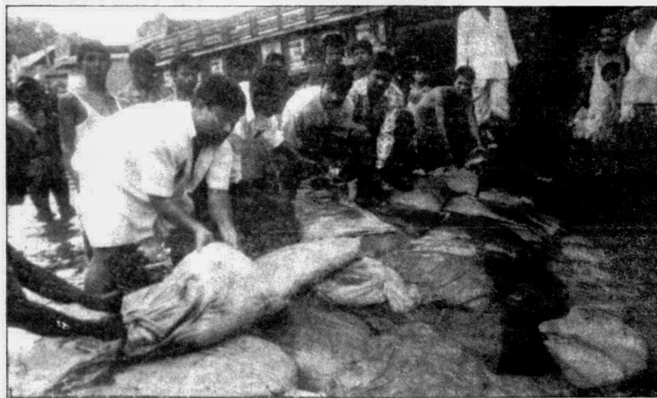
Mending the breach of Postagola embankment
