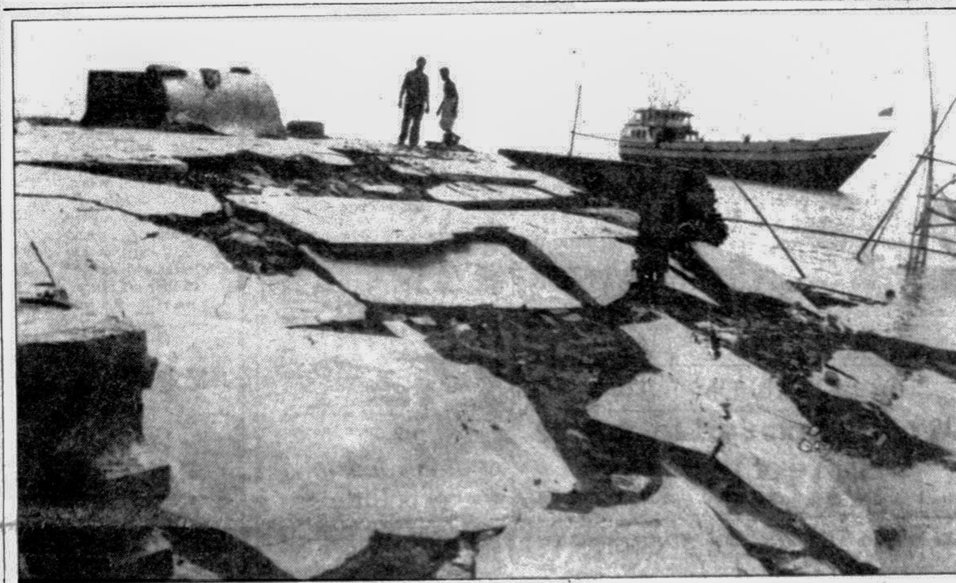
A flood-godown collapsed in flood and erosion in Ghoradour Union under Lohajang thana. — Star photo
