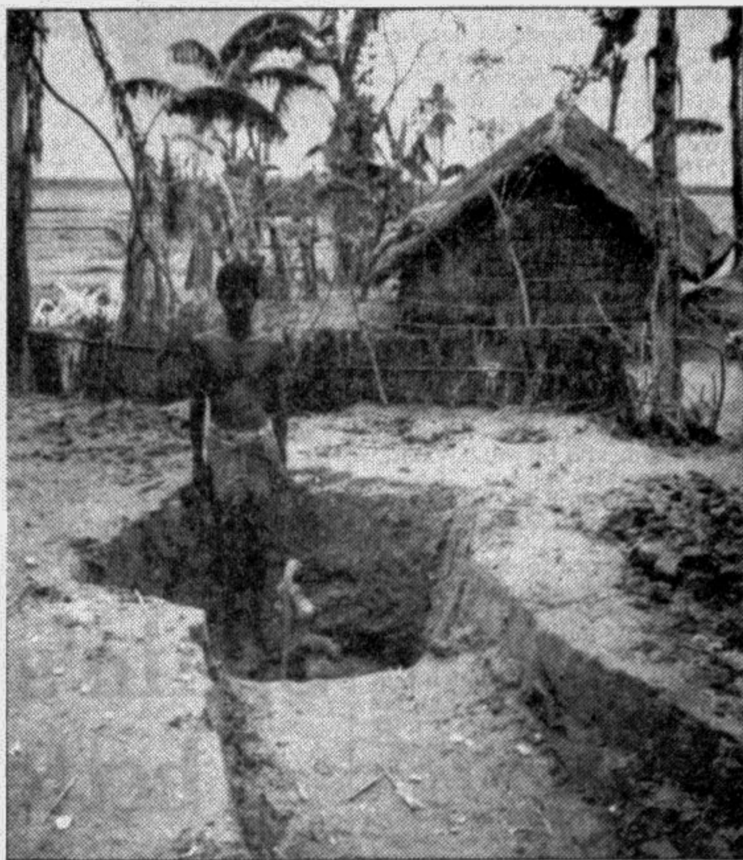
Villagers dug ten feet to reach the tubewell buried by silt during the flood. — Photo courtesy: BELA
