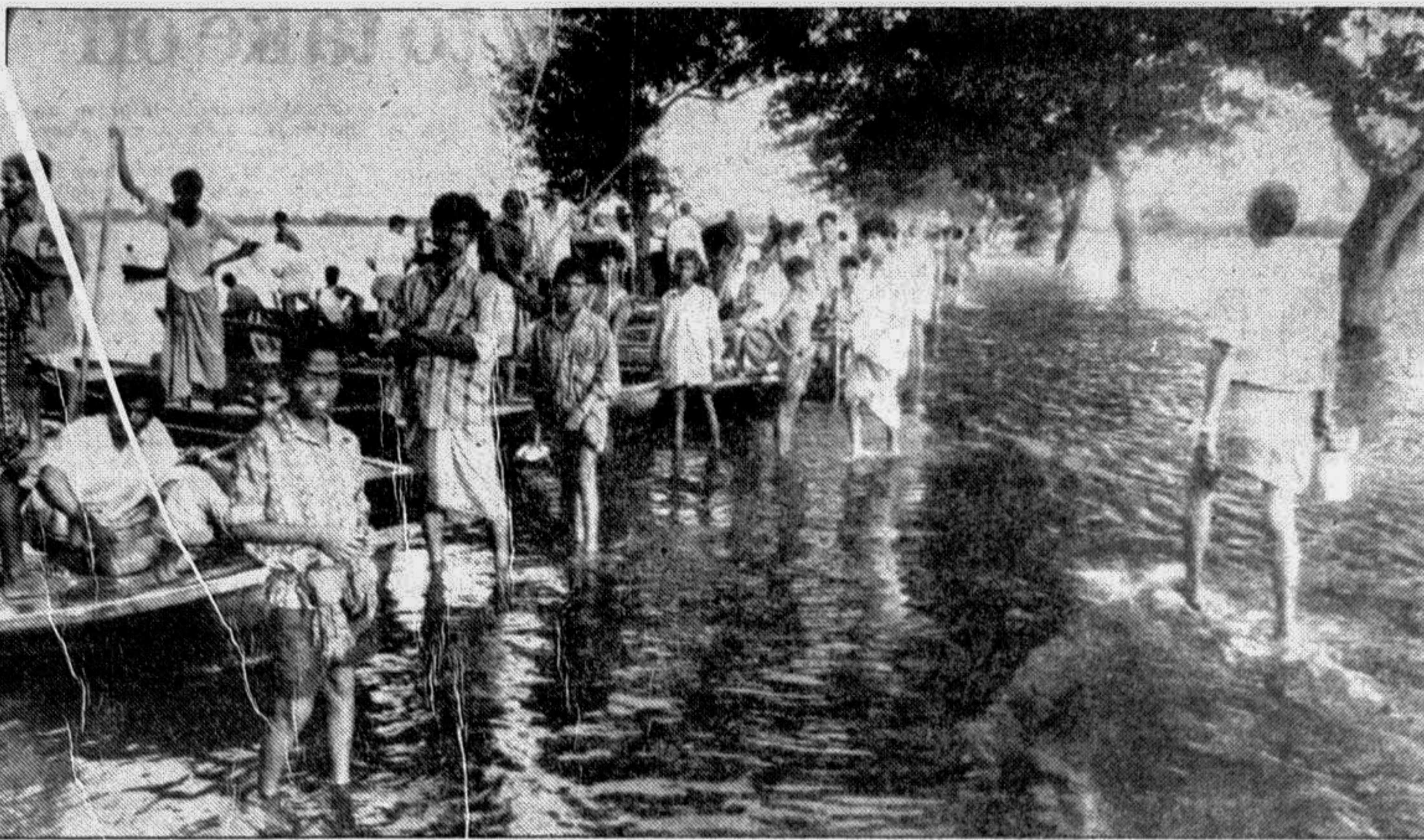
Dhaka-Chittagong Highway: Over flooded at Sonargaon area
