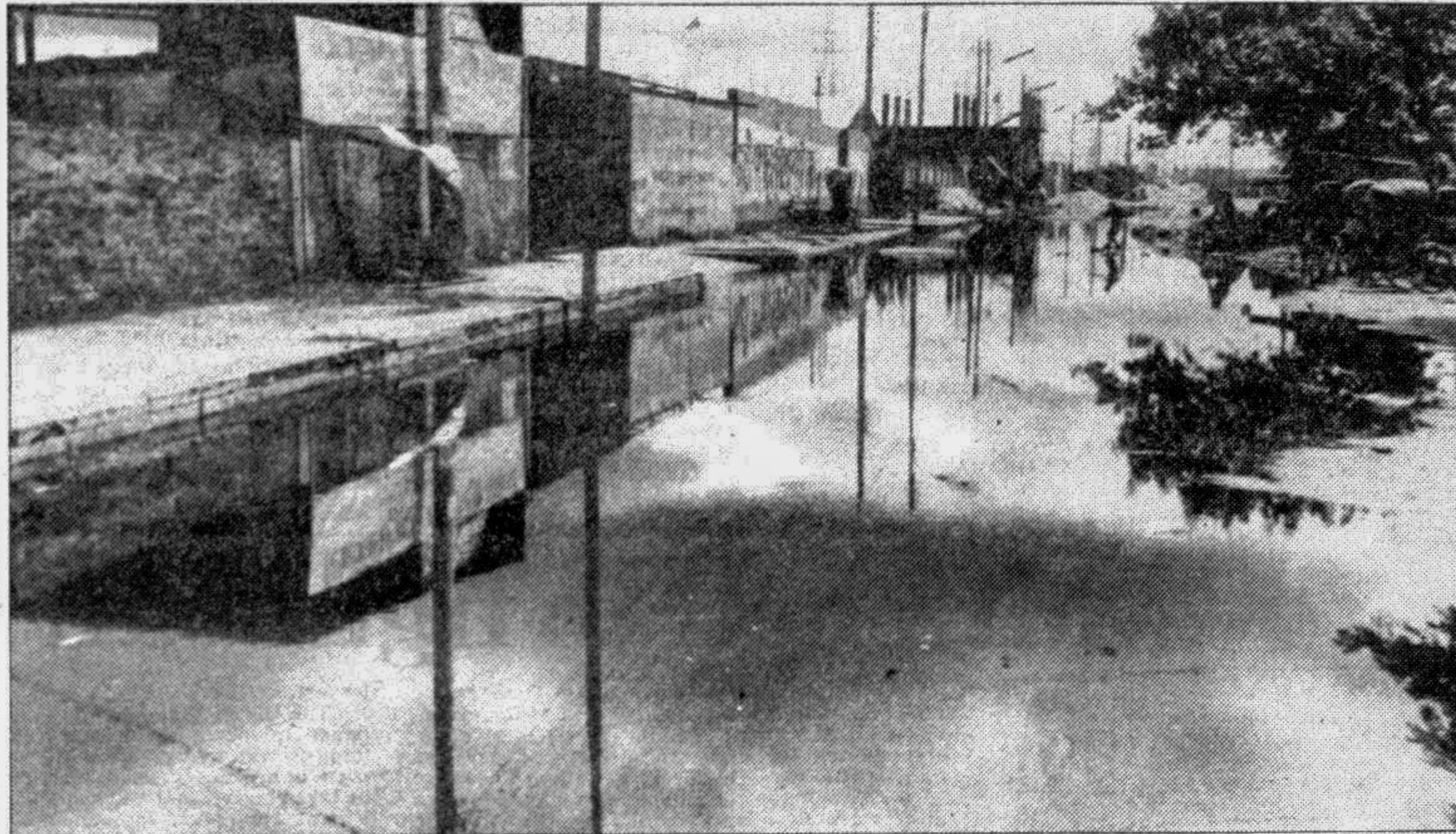
Floodwater seeping and submerging supposedly protected Shyampur Dhaka Match Factory area
