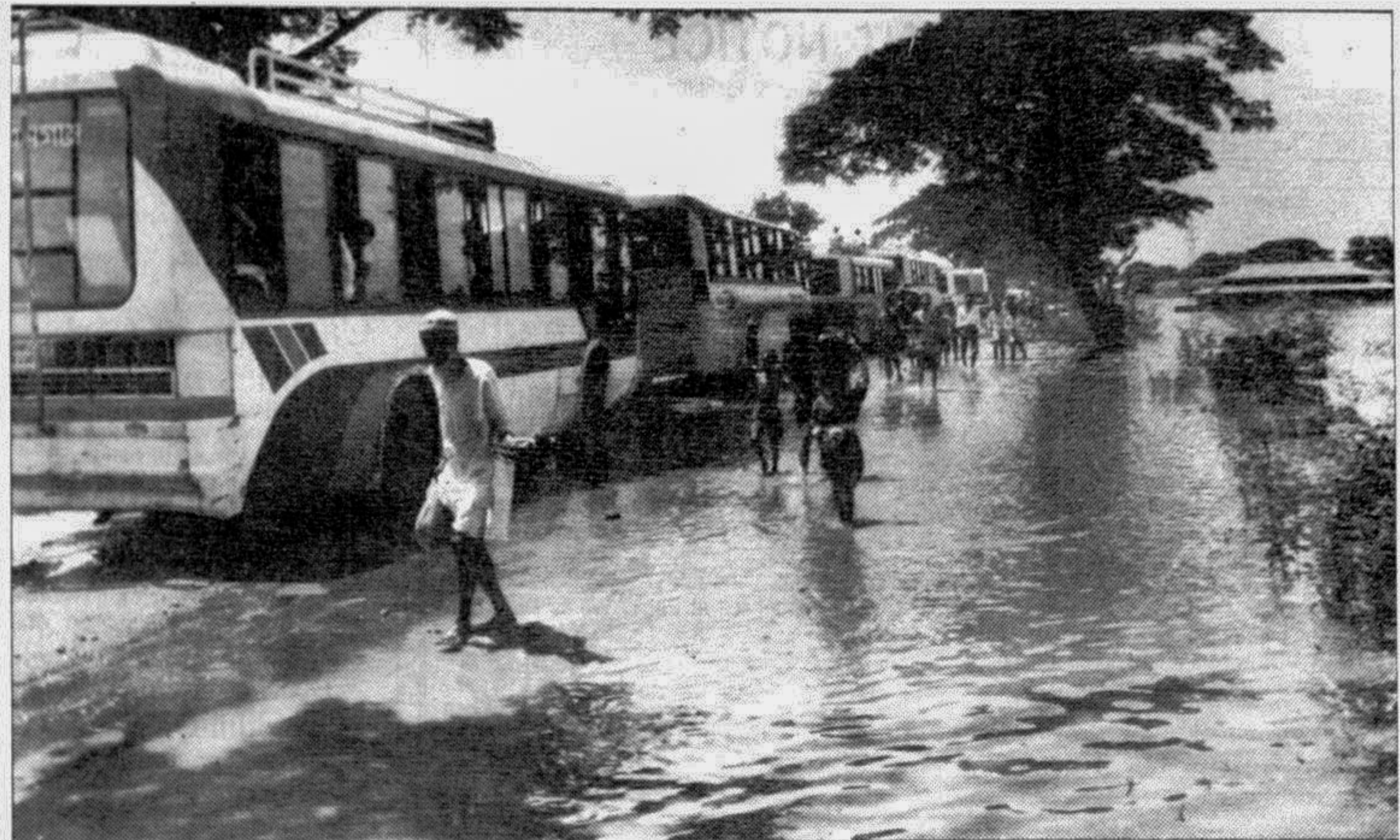
Traffic movement on Dhaka-Chittagong highway slowed down yesterday as flood water submerged the road near Jangla in Narayanganj thana. — Star photo
