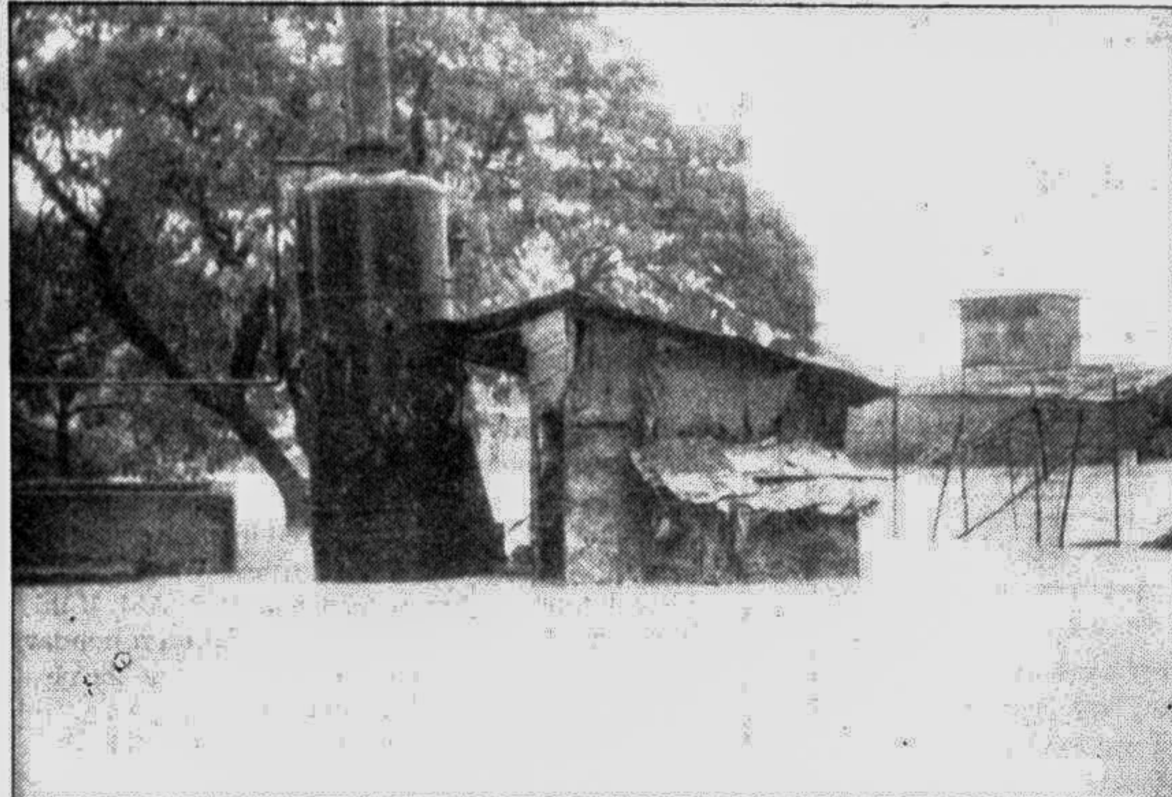
The water treatment plant at Kazirbazar in Sylhet town went under water as the Surma river is flowing above danger level. — Star photo
