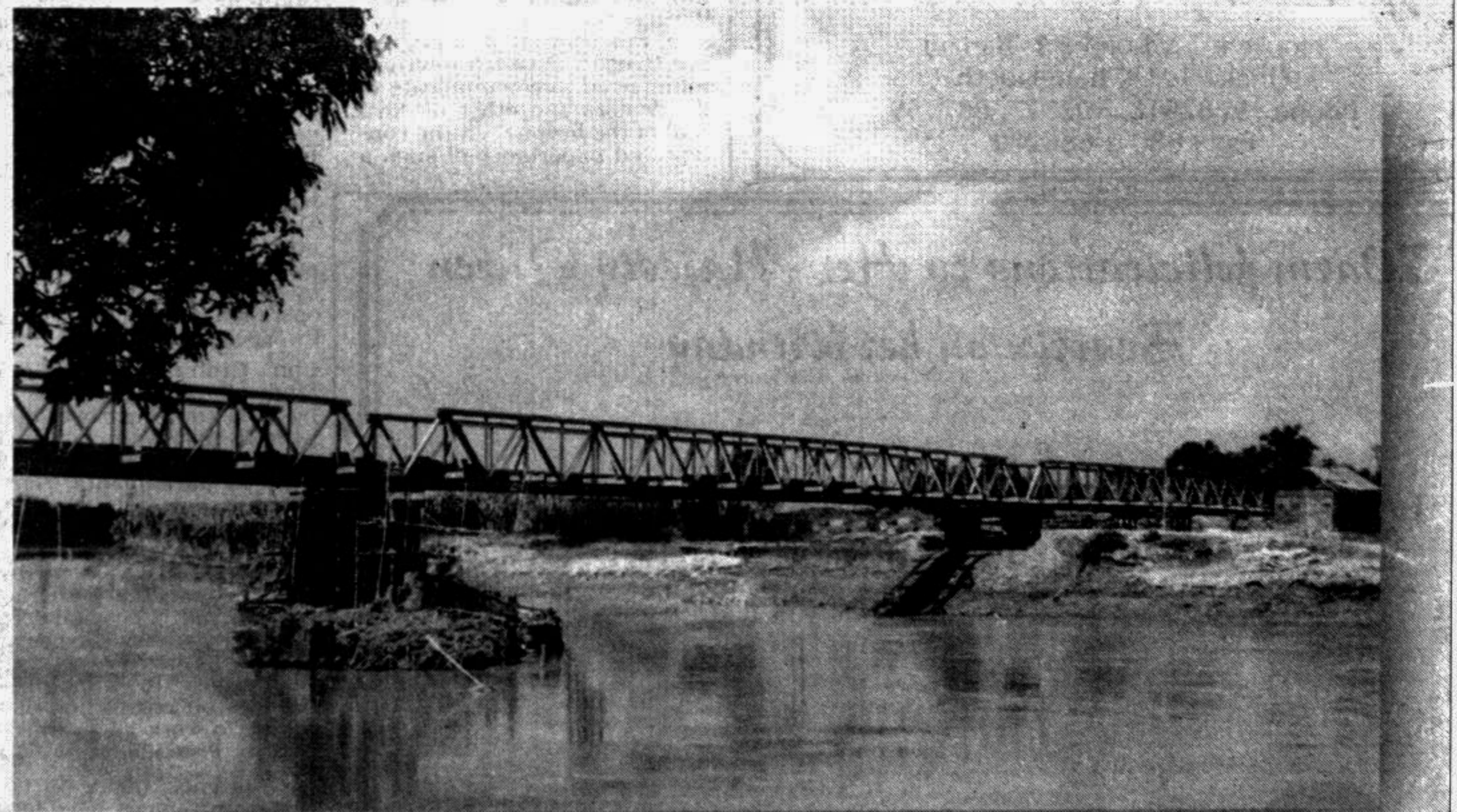
Newly erected Portable Steel Bridge (3x140 feet) in rural Bangladesh - designed, manufactured and supplied by Janson Bridging
