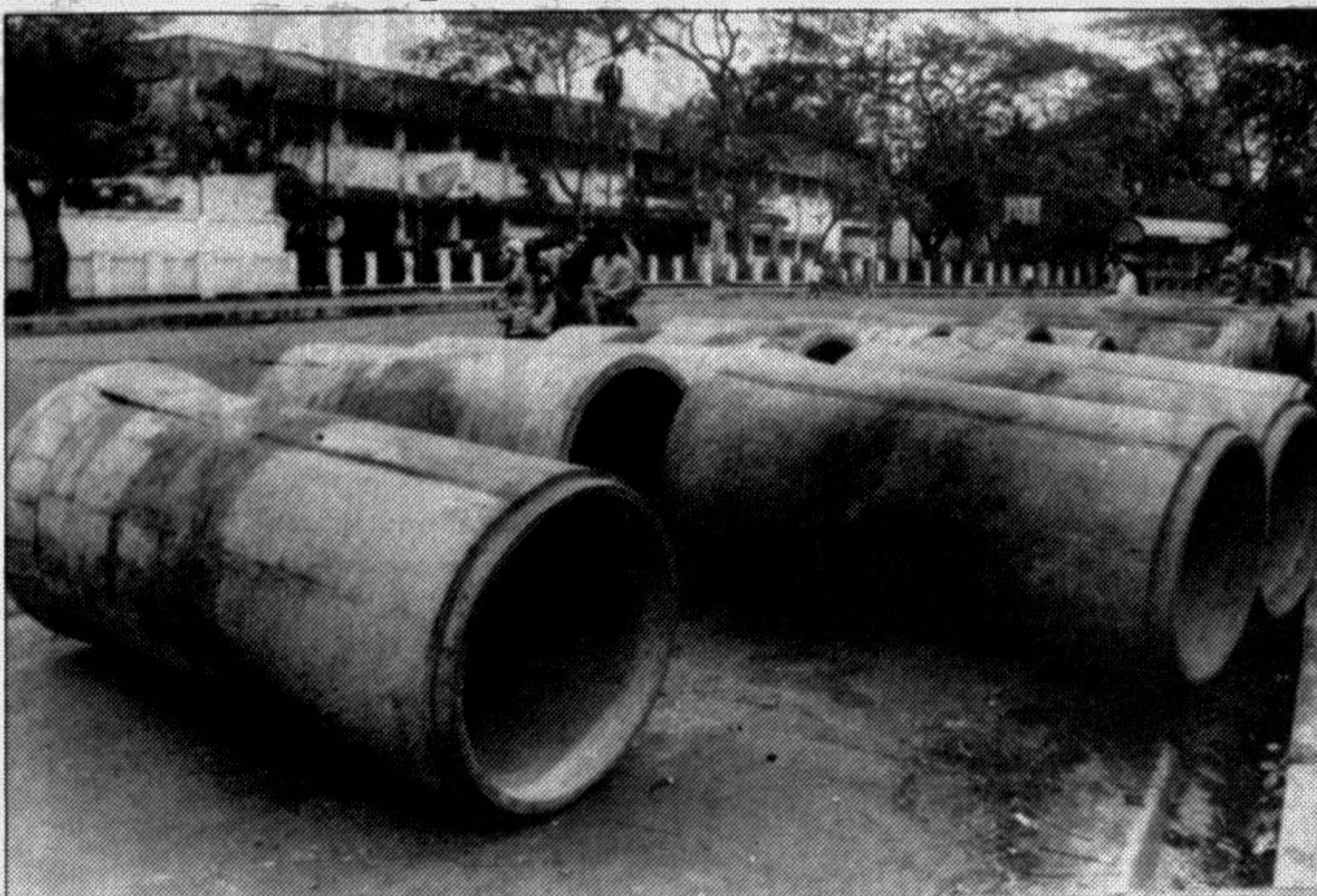
IF THE PIPES ARE HERE CAN MONSOON BE FAR BEHIND! Sewerage pipes are being stacked in front of the Dhaka University Arts Building. Soon the road will be dug up by concerned authorities with right earnest and rain will start falling, making life miserable for the road users. This, however, is the normal practice in Dhaka city. - Star photo
