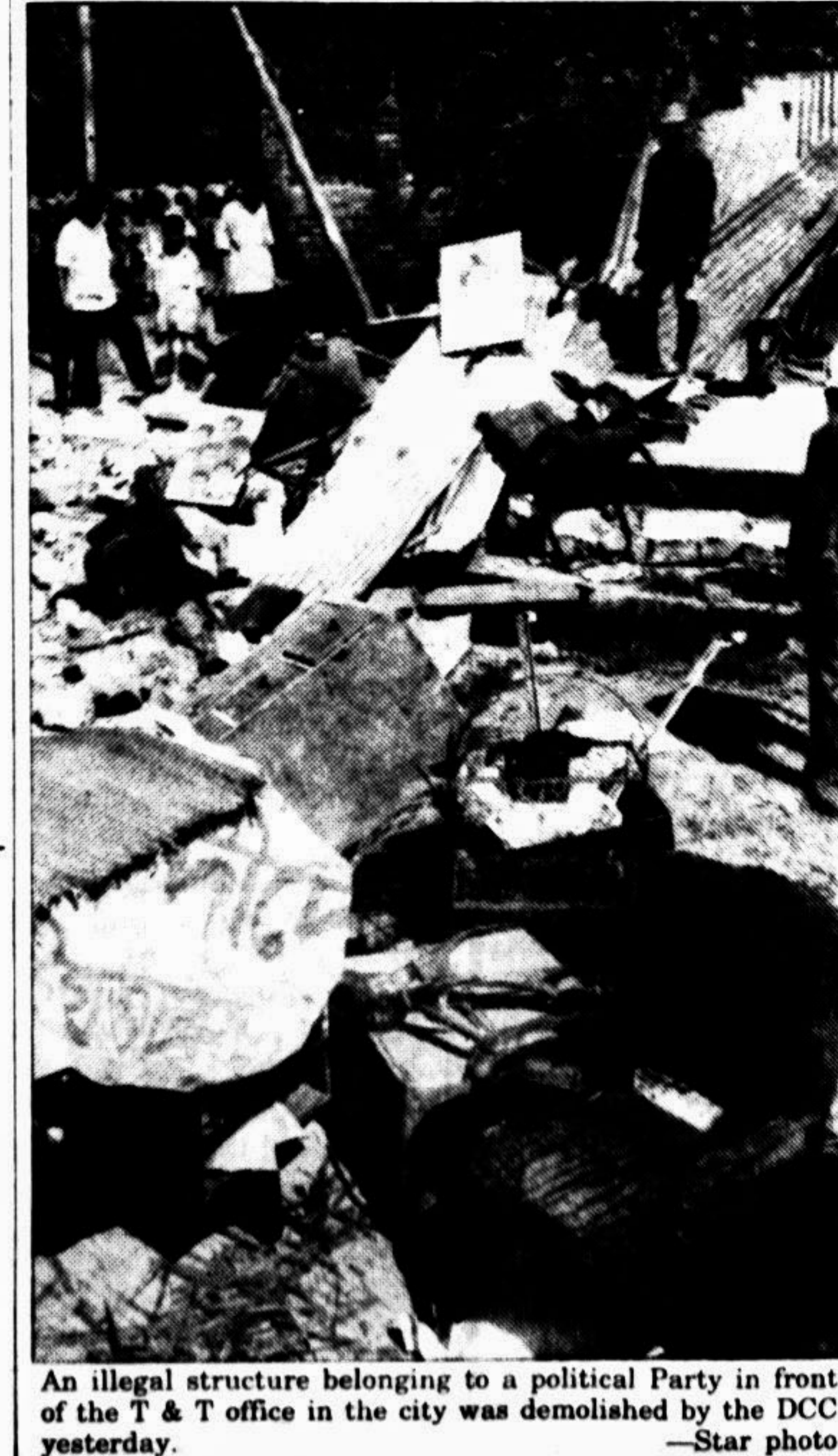
An illegal structure belonging to a political Party in front of the T & T office in the city was demolished by the DCC yesterday. —Star photo
