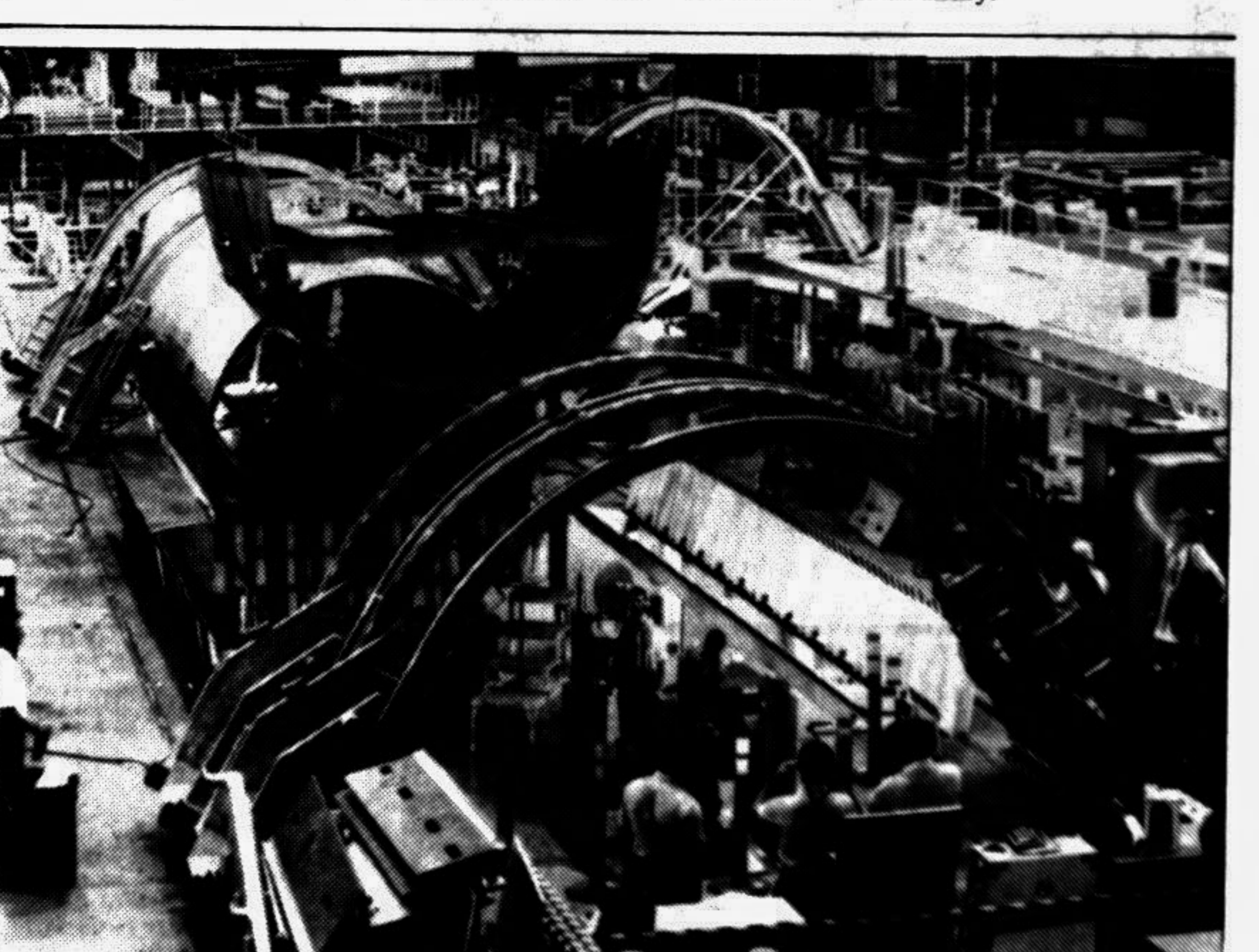
FIRST NEXT-GENERATION 737-600 FUSELAGE JOINED IN WICHITA: Workers at The Boeing Company's commercial division in Wichita, Kan., this month joined into one piece the major assemblies that comprise the fuselage of the first Next-Generation 737-600 airplane. Photo shows the Section 43 lower lobe as it is being lowered into an integration tool for joining. After integration of the fuselage is complete, protective finishes will be applied and the unit will be shipped by rail to the company's commercial division in Renton, Wash., where final assembly and delivery will take place. Smallest of the Next-Generation 737 family, the -600 model measure 110 feet 4 inches (31.2 m) in length and can carry up to 132 passengers. The 737-600 was launched in 1995 by Scandinavian Airlines System (SAS) when the airline ordered 35 of the aircraft. The first 737-600 will roll out of the Renton factory in December 1997. First flight is scheduled for January 1998 and delivery is set for August of next year.
