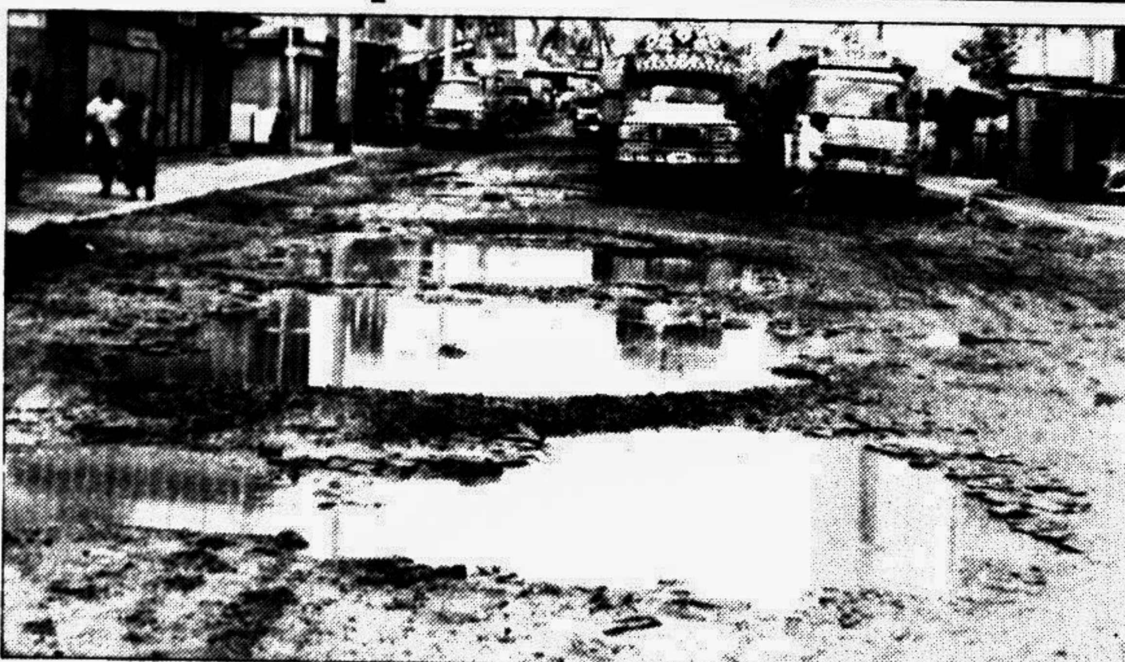
Potholes in Kwaran Bazar road in the city.
