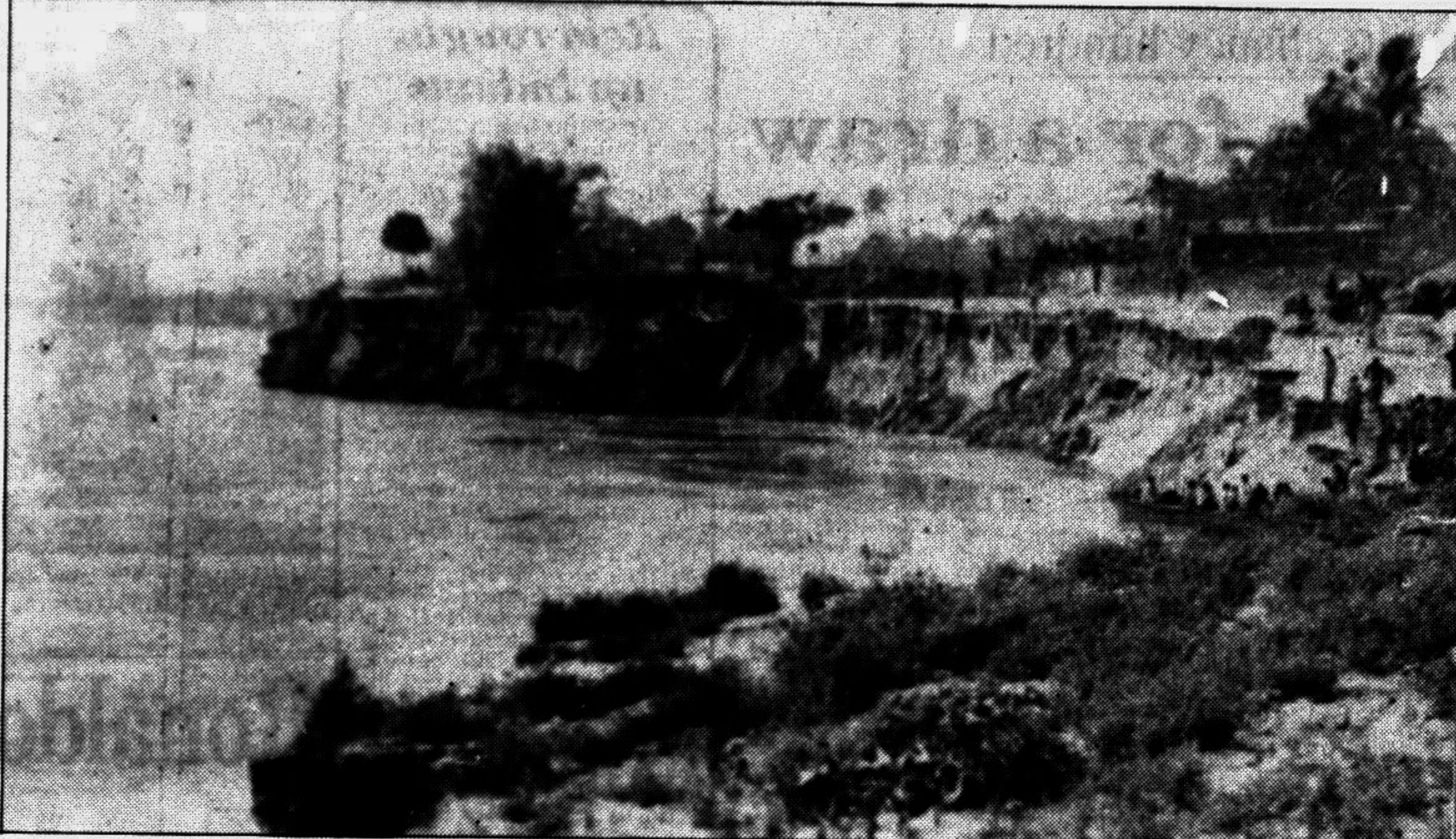
GAIBANDHA : About 300 families of two villages namely Chakuli and Bangabari under Shaghata thana in the district have been rendered homeless by erosion of the river Katakhal due to sharp fall in its water level in last few days. The two villages are on the verge of extinction now. Nine more villages such as Ramnagar, Kachua, Chandanpat, Kingkorpur, Jamalair, Pakurtola, Panchpur, Simulbari and Bolierbar are also affected by the river erosion. Yet no step has been taken by the authorities to contain the erosion. Out of total 300 erosion affected families, 100 families passing their days under open sky and the remaining families have taken shelter in different educational institutes of the area. The photo was taken recently by our local correspondent K M Rezaul Haque.
