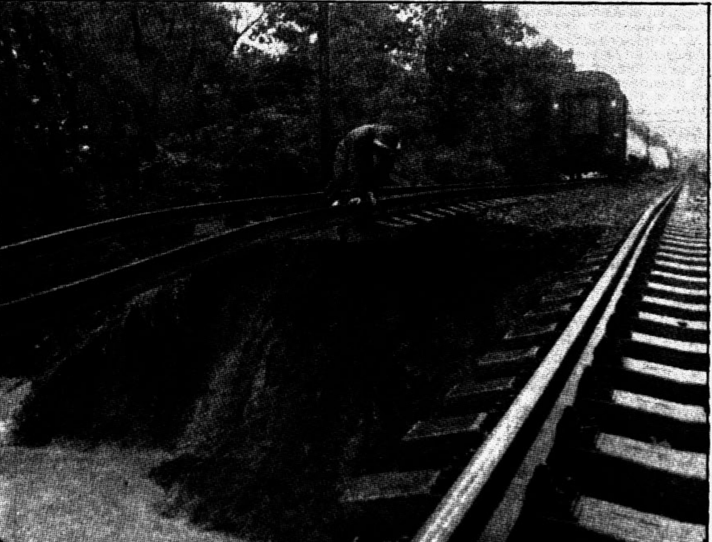
A man inspects Tuesday the rails damaged by swollen water near the spot where an express train (background) en route from Vienna to Warsaw derailed Monday near Suchdol nad Odrou. Workers at the spot are still not able to remove the damaged train as the area is still flooded after several days of heavy downpour. — AFP/UNB photo
