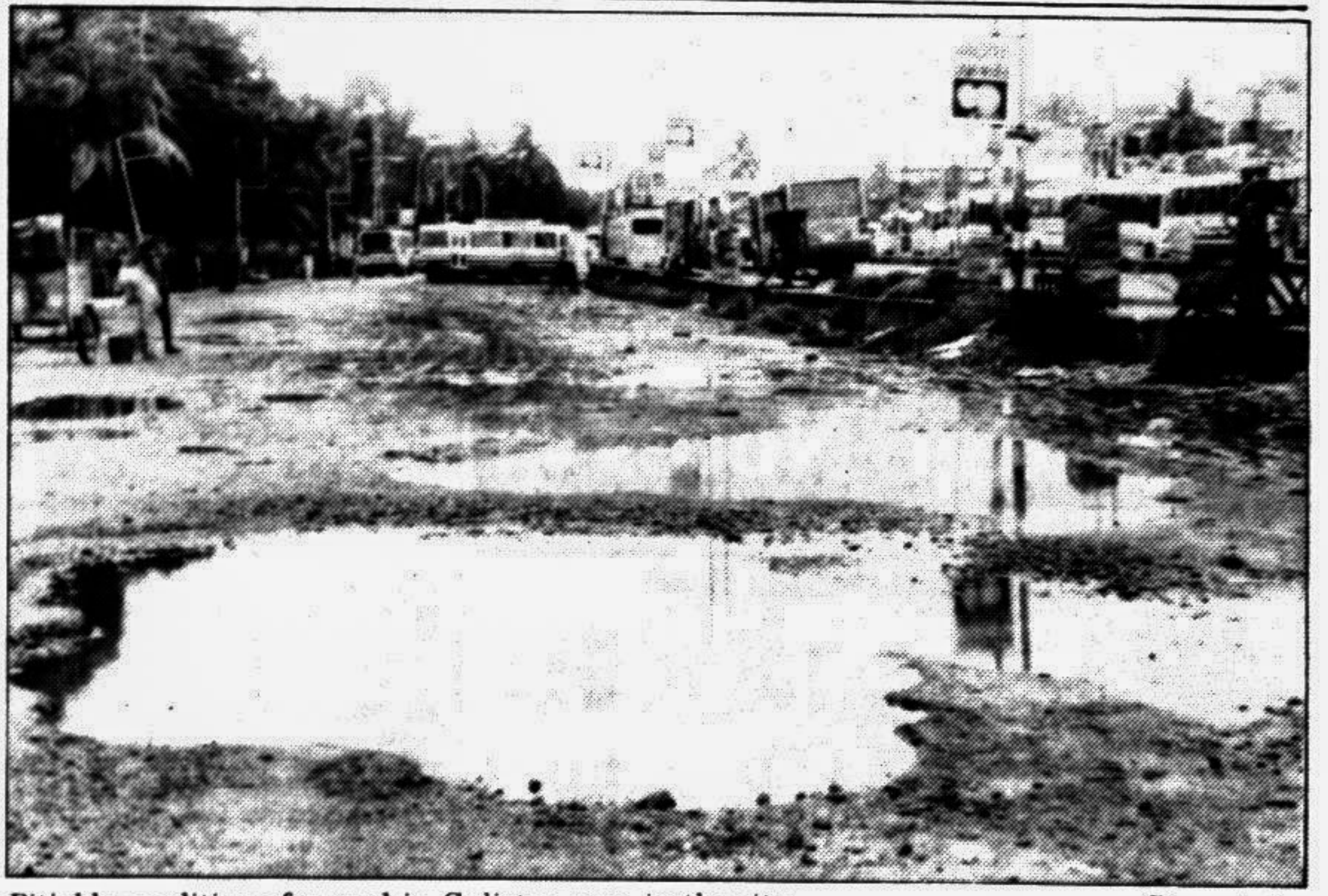
Pitiable condition of a road in Gulistan area in the city. —Star photo
