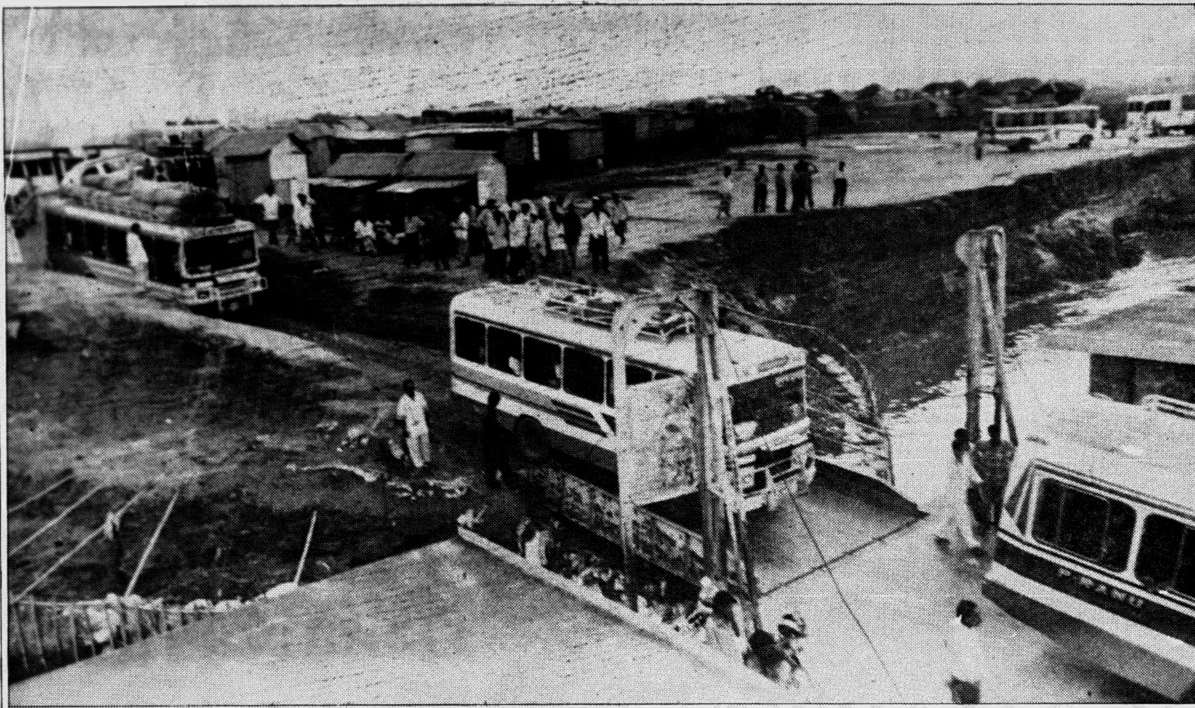
Dhaka-Mawa road, a short distance highway through Bhanga thana of Faridpur constructed to reach destinations in south and south-western districts has been threatened by Padma river erosion at the Mawa ferry ghat point. This picture shows Mawa ferry ghat point. It shows embankment near the pontoon already experiencing erosion threatening business establishment at the ghat as well as the road linking the pontoon.
