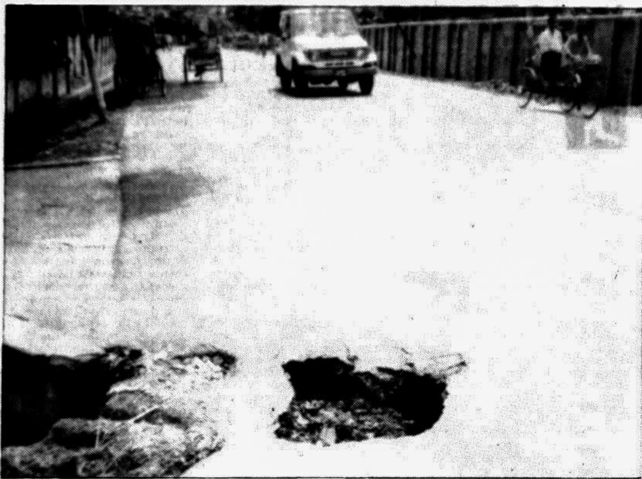
PABNA: Potholes on an important road in the town. The road was developed at a cost of huge amount of money a few months back. Within a short span of its construction cracks and potholes developed on the road posing threat to the passers-by as well as vehicles. Lapses in development works are behind creation of such situation. Attention of Pabna pourashava is drawn to look into the matter so that repetition of such negligence does not occur in future at the cost of hard earned people's revenue.— Star photo by Ranesh Maitra
