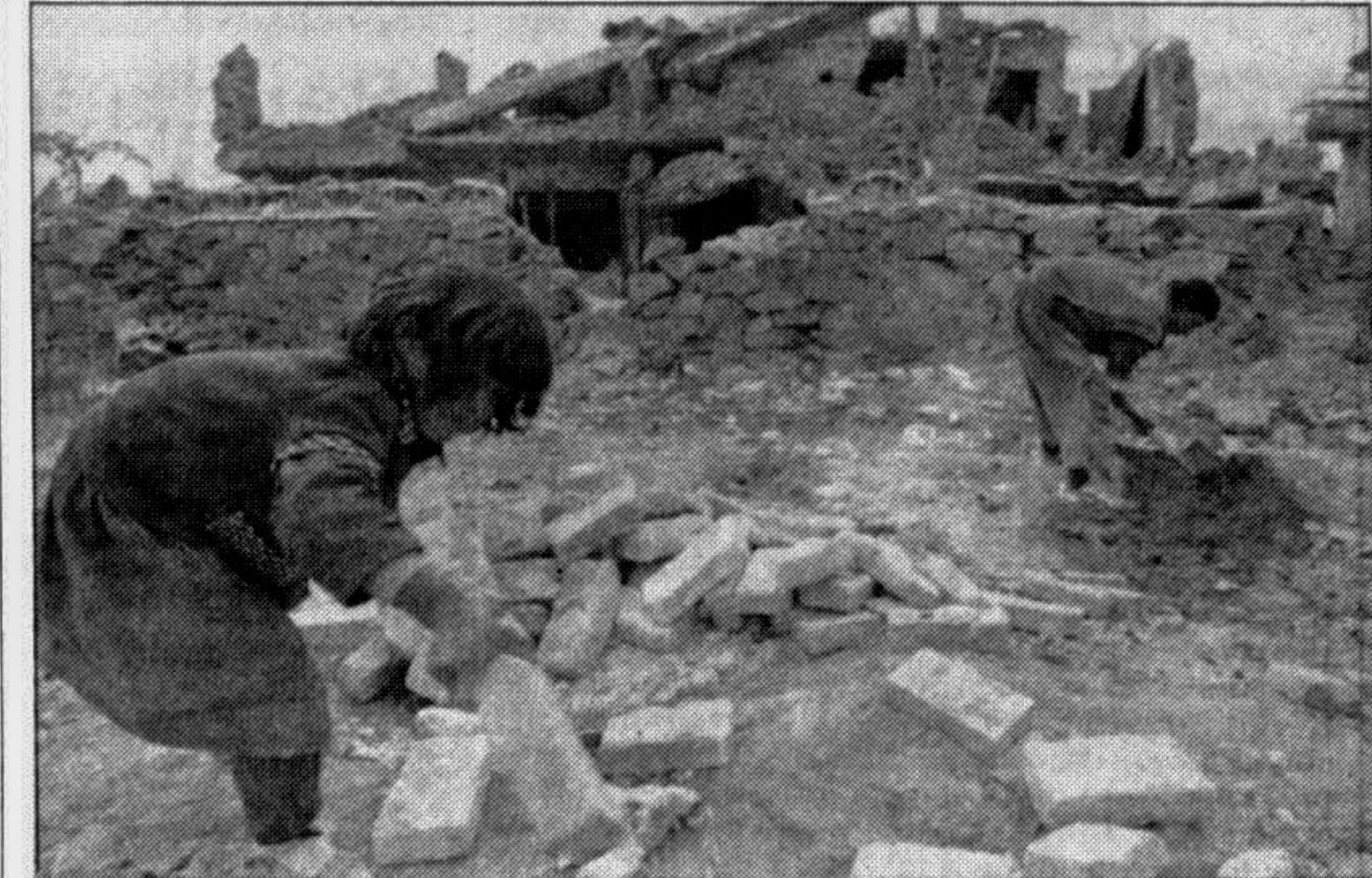
An Afghan girl (L) helps her brother by collecting bricks from the rubble for the construction of a small shop at Kar Tesi, south Kabul, in Afghanistan on Friday. The Kar Tesi area has been completely destroyed due to heavy fighting between the Afghan factions. — AFP/UNB photo
