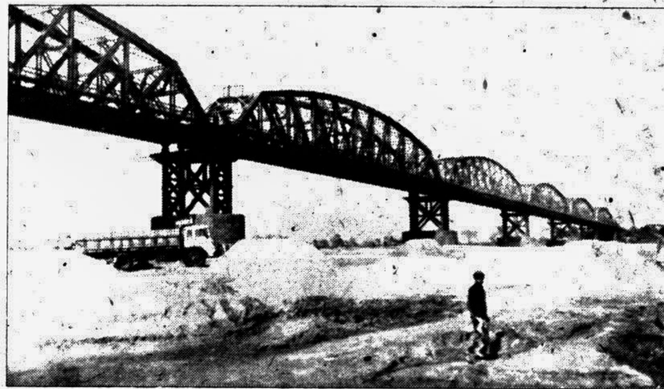
The dried up 'Padma' at Hardinge Bridge, Paksey
