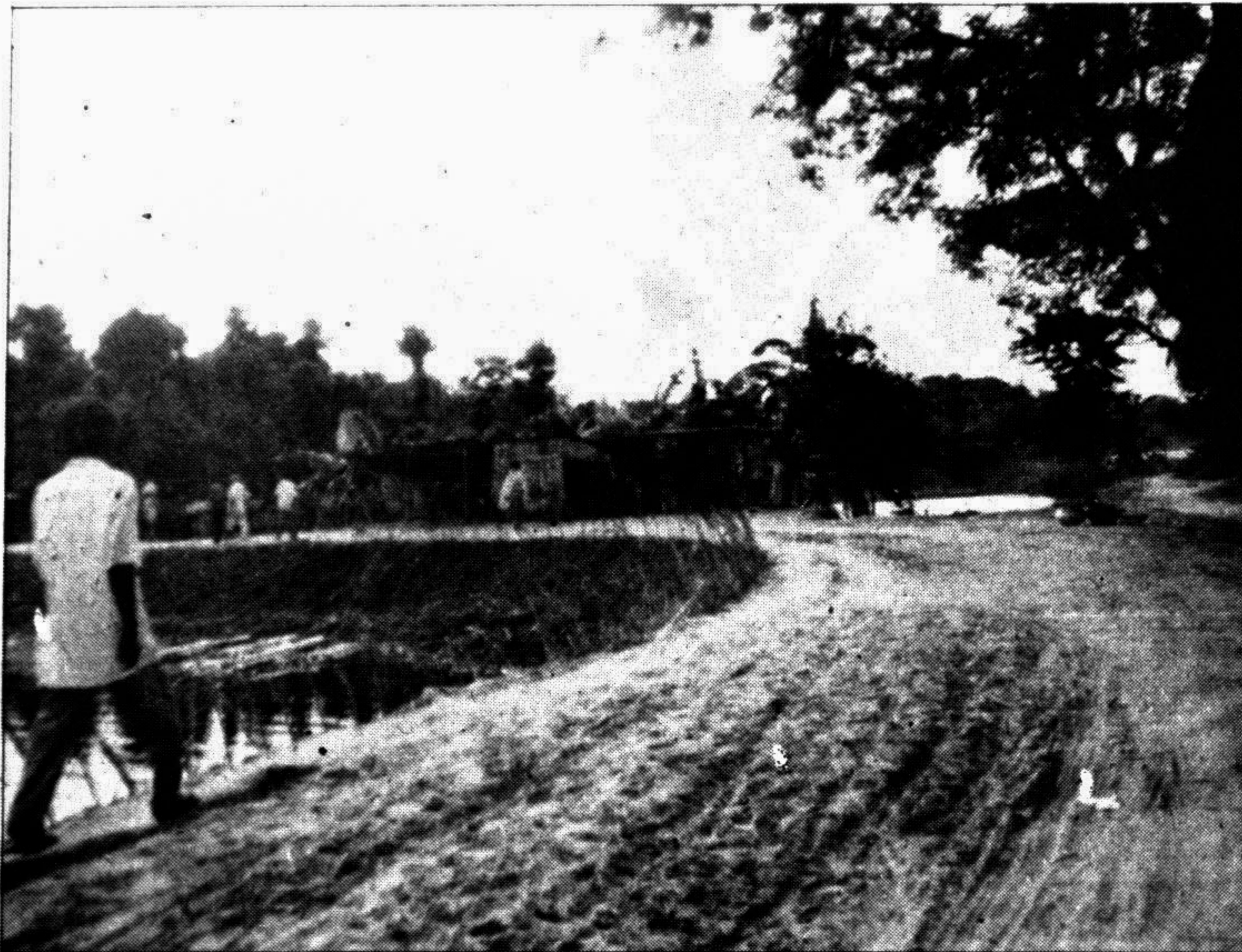
PABNA: The Baral river. An embankment constructed right through the river cut off water flow of the river. — Star photo
