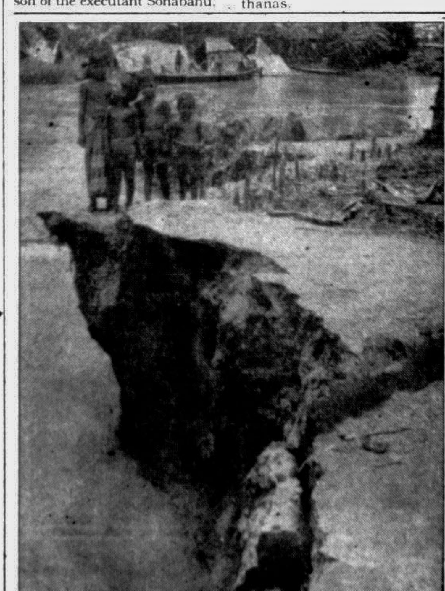
TANGAIL: Picture shows a bank in Kaku village, Tangail, under severe threat of erosion. — Star photo
