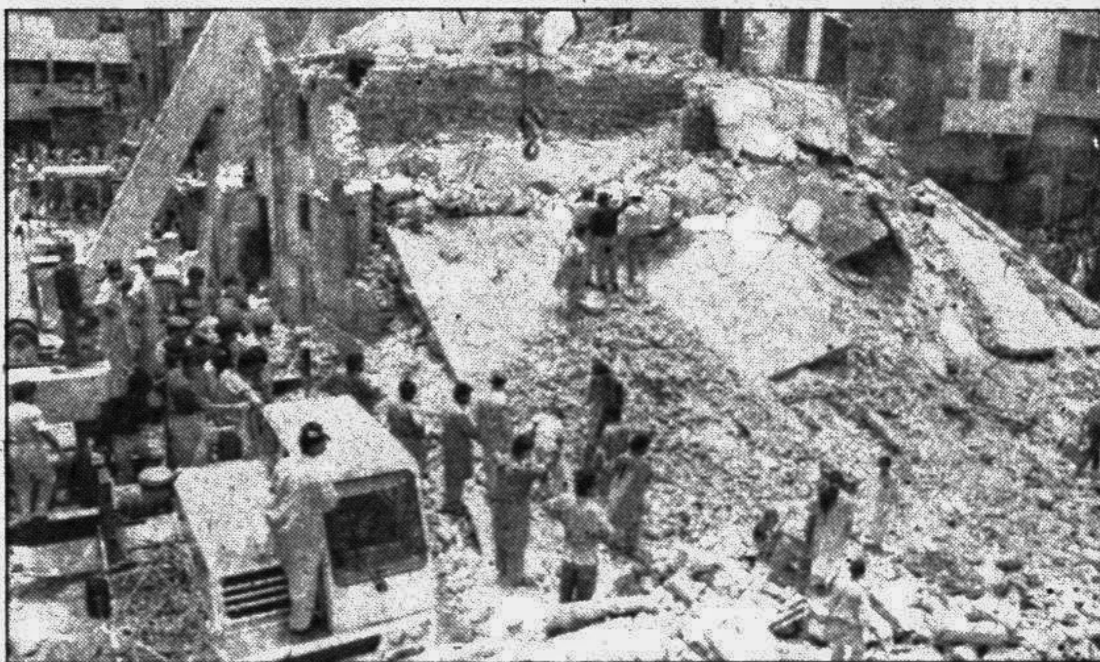
Rescue workers go through the rubble of the collapsed building to find out bodies in Hyderabad, some 160 Km from Karachi, Wednesday. At least 22 people were killed and 40 injured when a three-story building collapsed in the early hours. — AFP/UNB photo
