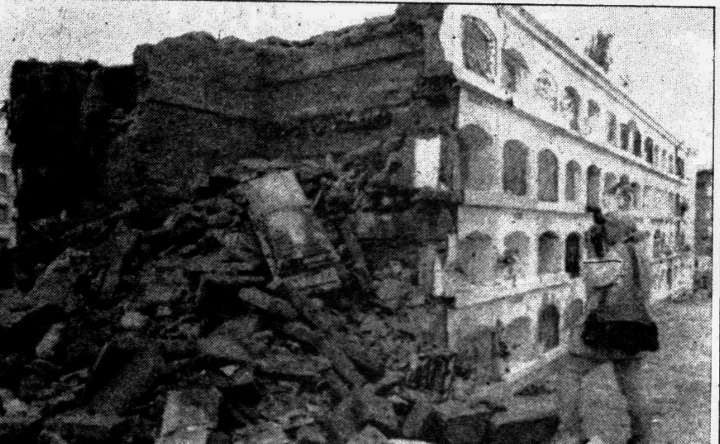
A press photographer takes pictures on Friday of the Pujili cemetery partially destroyed by a late Thursday earthquake which reportedly destroyed some 200 homes in the town south of Quito, Ecuador.
