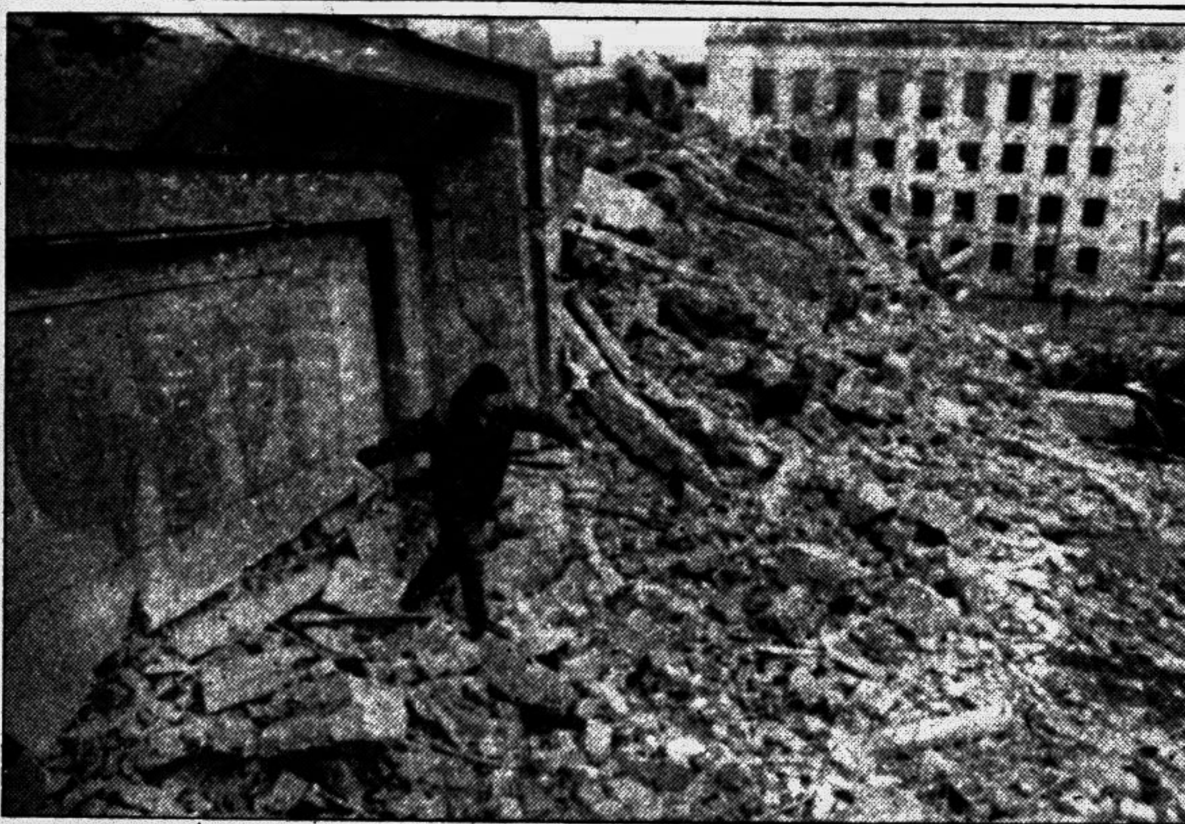
A man steps on the rubble surrounding the ruins of the Presidential palace in Grozny on Saturday. The palace building was blown up last week by Russian forces. The pro-Russian Chechen government took steps on Sunday to prevent new mass demonstrations by separatists by not authorising demonstrations February 23 when Chechens observe the anniversary of their mass deportation by Stalin in 1944. — AFP/UNB photo
