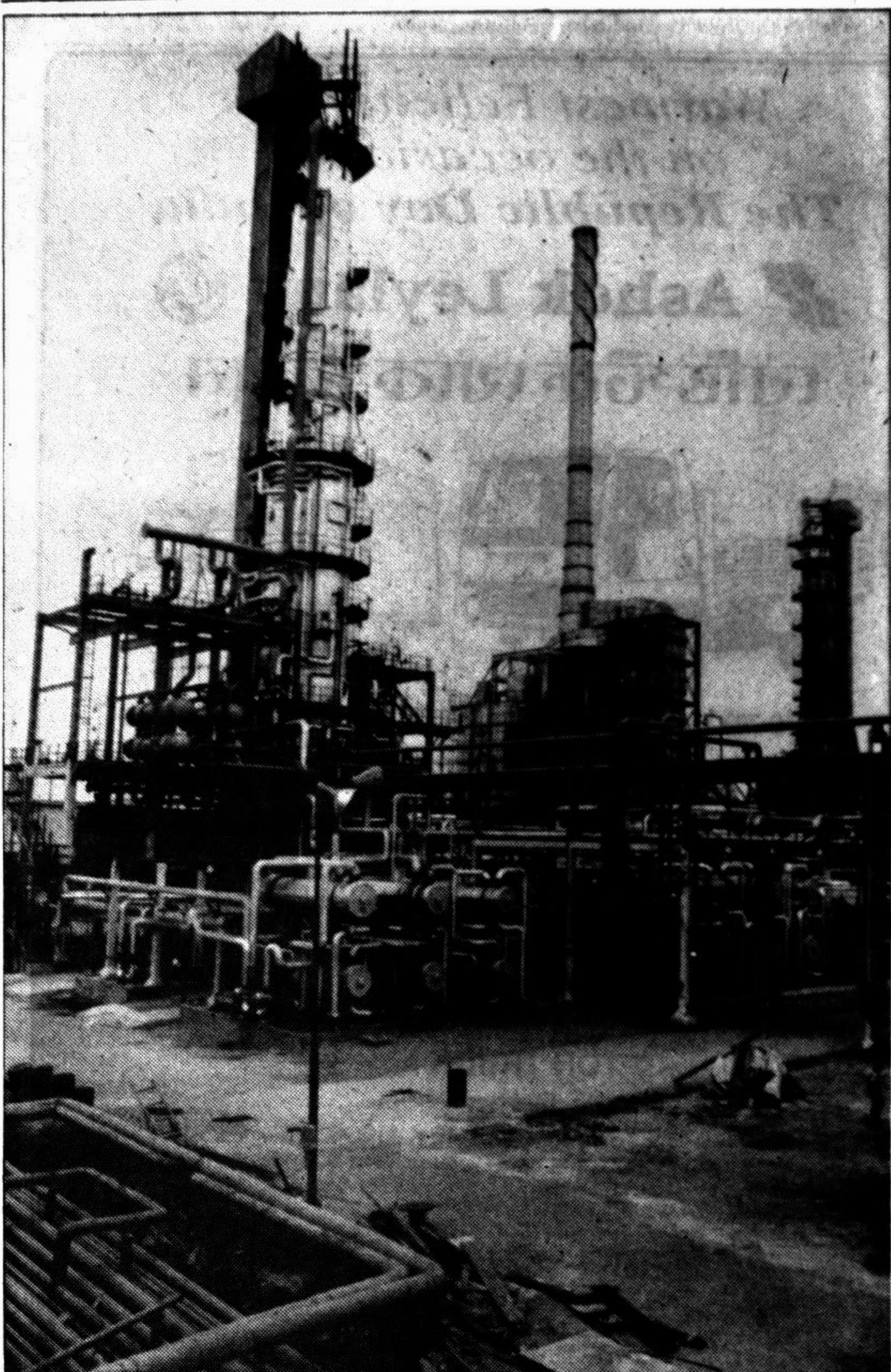
A close-up of the new primary grade distillation tower and furnace at HPC's Bombay Refinery
