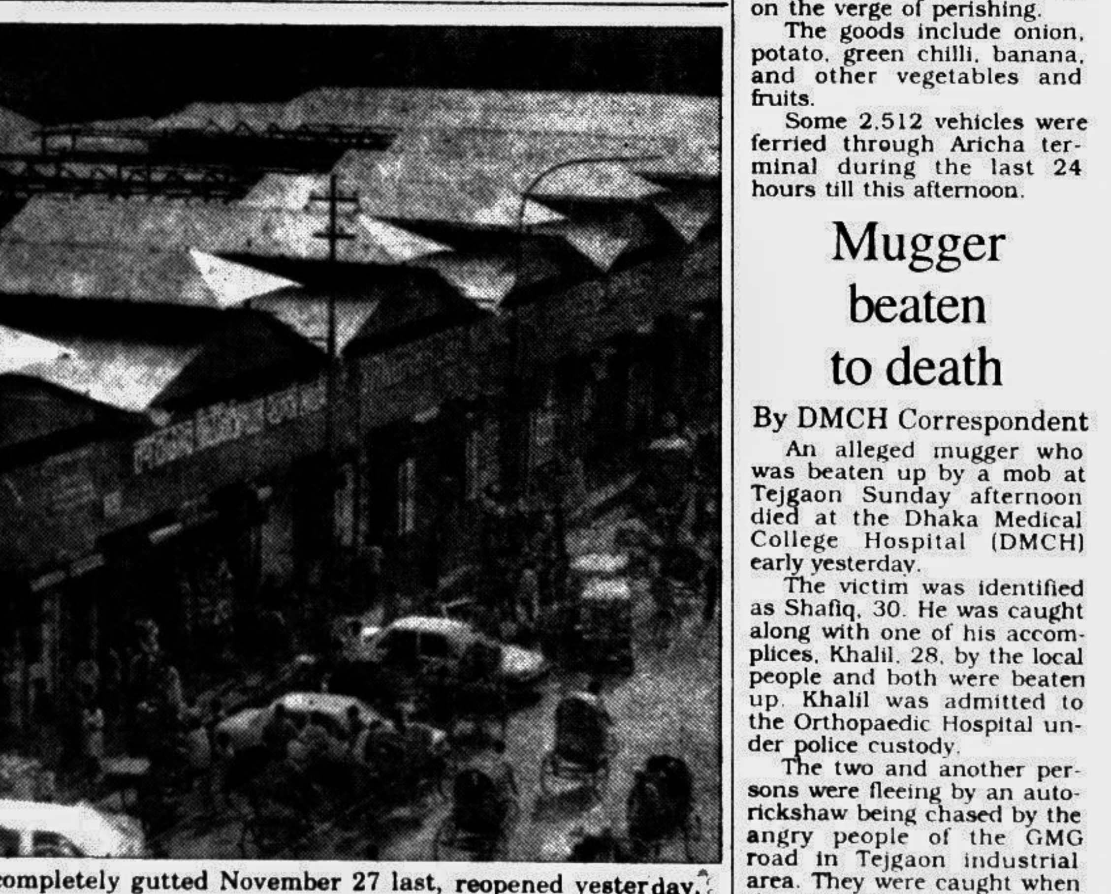
The Bangabazar, which was completely gutted November 27 last, reopened yesterday. — Star photo
