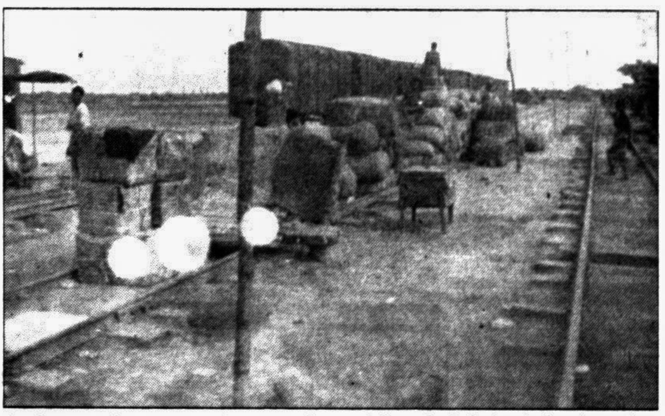
Goods meant for transportation across Jamuna left at the Bahadurabad train station. Ferry services at Bahadurabad ghat remain suspended causing untold sufferings.
