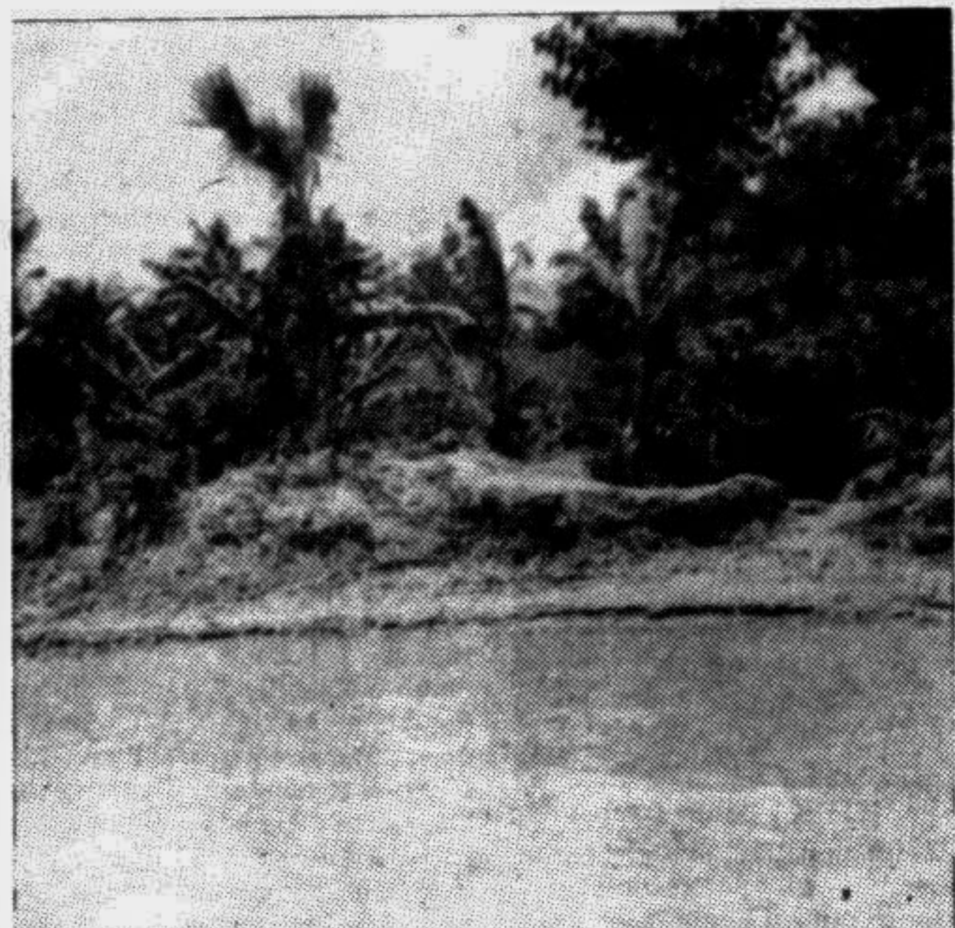
PABNA: The picture shows erosion affected Nagarbari ferry ghat. In near future erosion may take more severe turn, it is apprehended by the people living around Nagarbari. — Star photo
