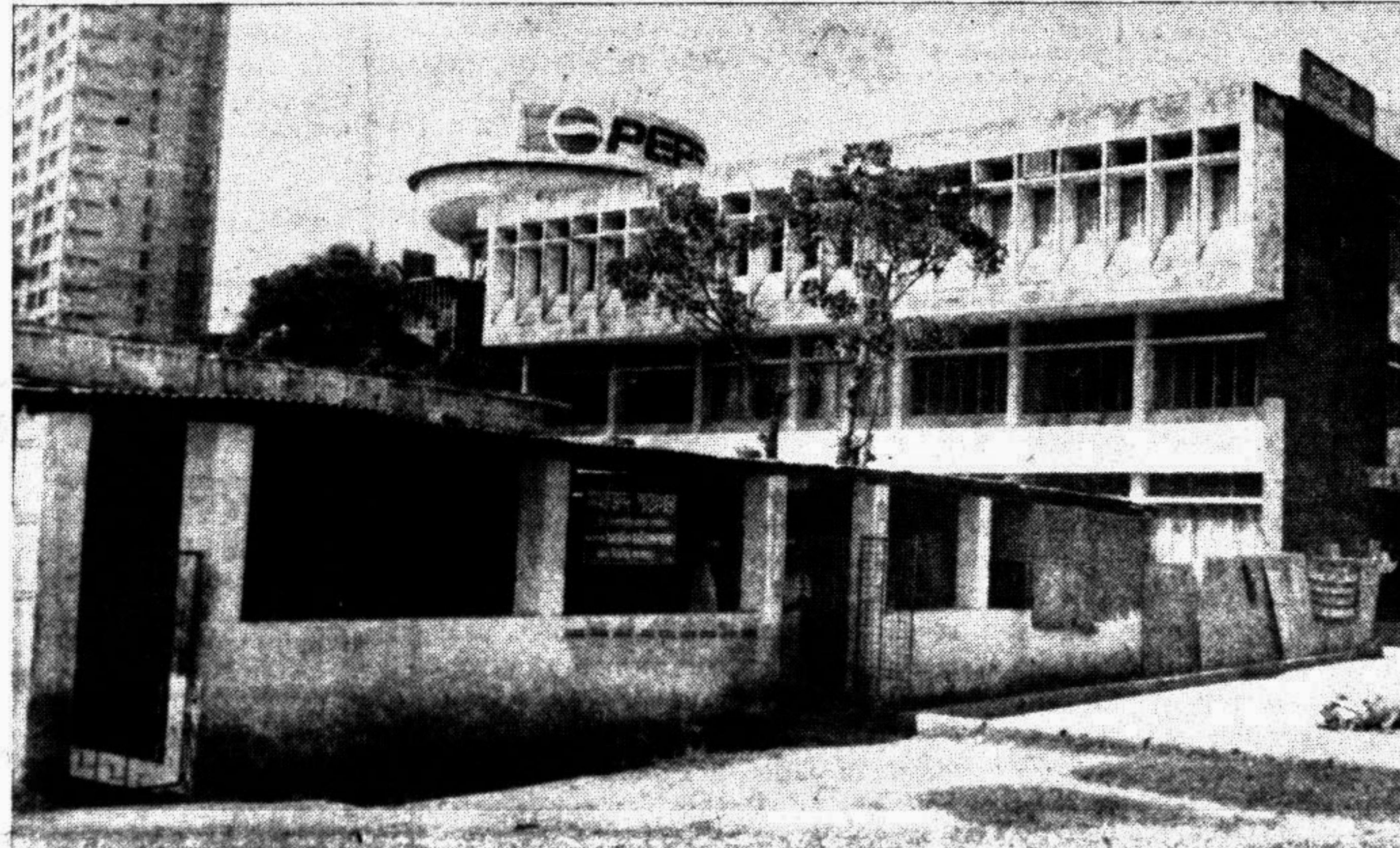
An unauthorised construction inside the Cancer Research Institute premises at Mohakhali in the city. — Star photo
